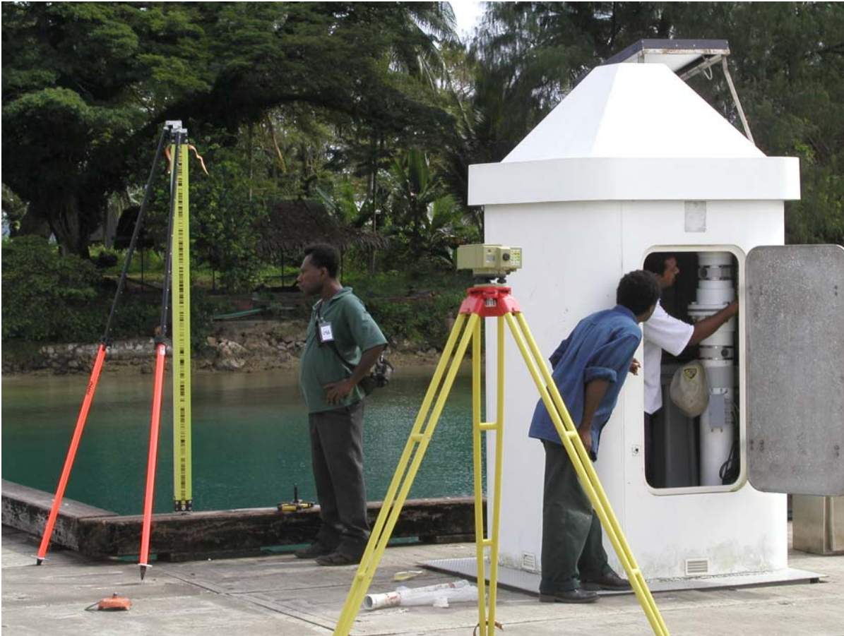
The Tide Gauge on the Lumbrum Wharf at the Manus Island in Papua New Guinea with the surveying equipment (Digital Level & Invar Bar Coded Staff) in the foreground. In this photograph are Andrick with Joe and Alsoi of the Survey Department of PNG checking on the Tide Gauge.
