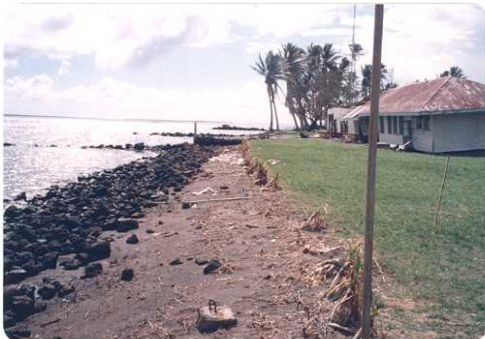
Figure 19. Coastal erosion on the lagoon facing, northern point of Mulinu'u Peninsula was significant.
