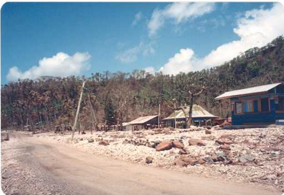
Figure 27. Power lines at Lautuanuu Village were severed when waves knocked the poles from their foundations and high winds severed the electrical lines.
