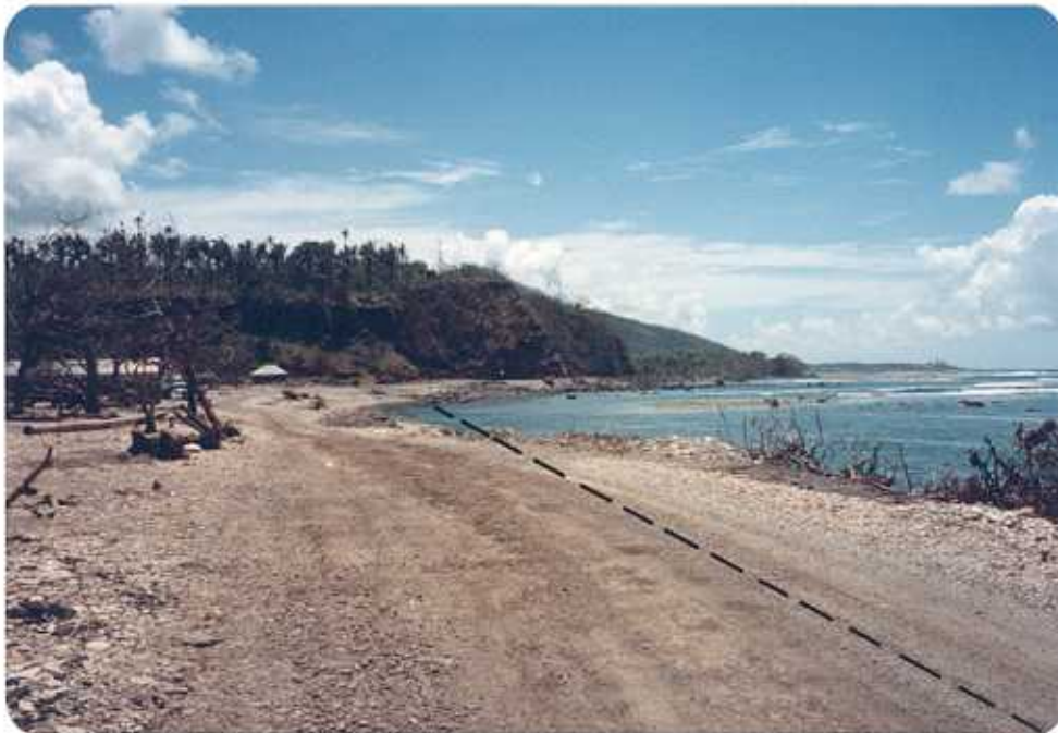
Figure 22. At Lautuanuu Village the road was completely washed away disrupting travel to the east of Apia and hindering rescue operations after the cyclone. The original road lay along the dashed line in the photograph.
