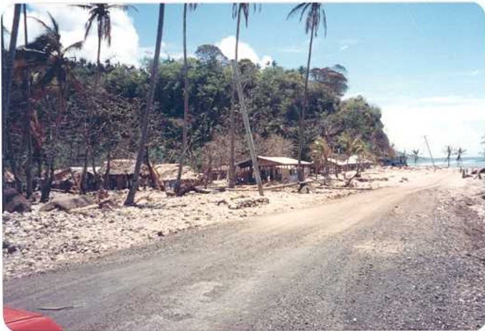
Figure 4. Destroyed homes and power lines at Lautuanuu Village. The road lies next to the coastline. Coral rubble now covers areas that were carefully tended lawns and gardens.
