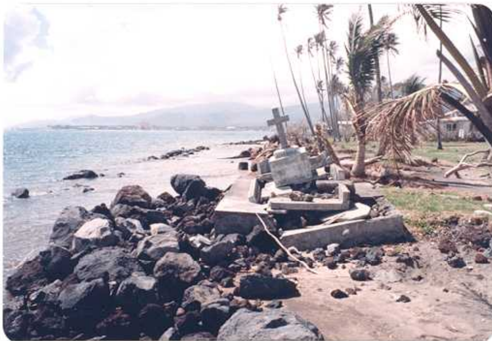
Figure 21. A grave site lying along the coast on the east side of Mulinu'u Peninsula survived the cyclone with little additional damage due to the placement of a protective rock fill in December, 1990 which absorbed much of the wave energy expended on the coastline. The rocks from the fill can be seen scattered around the site. These coastal monuments were considered by Carter (1987) to be at high risk during a cyclone.
