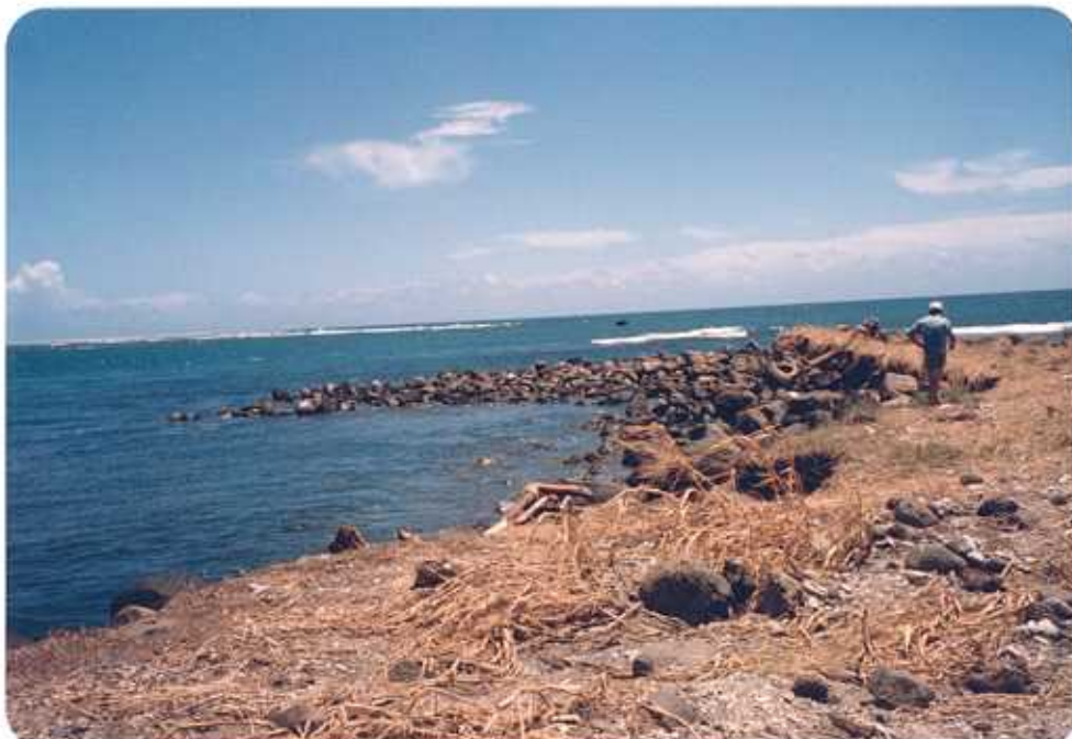
Figure 32. The loss of reclaimed land was significant along the entire northern coast of Upolu. The landfill area in this photograph lies directly off the city front in Apia and about 20 meters of the ocean fronting portion was lost to wave attack during the cyclone.
