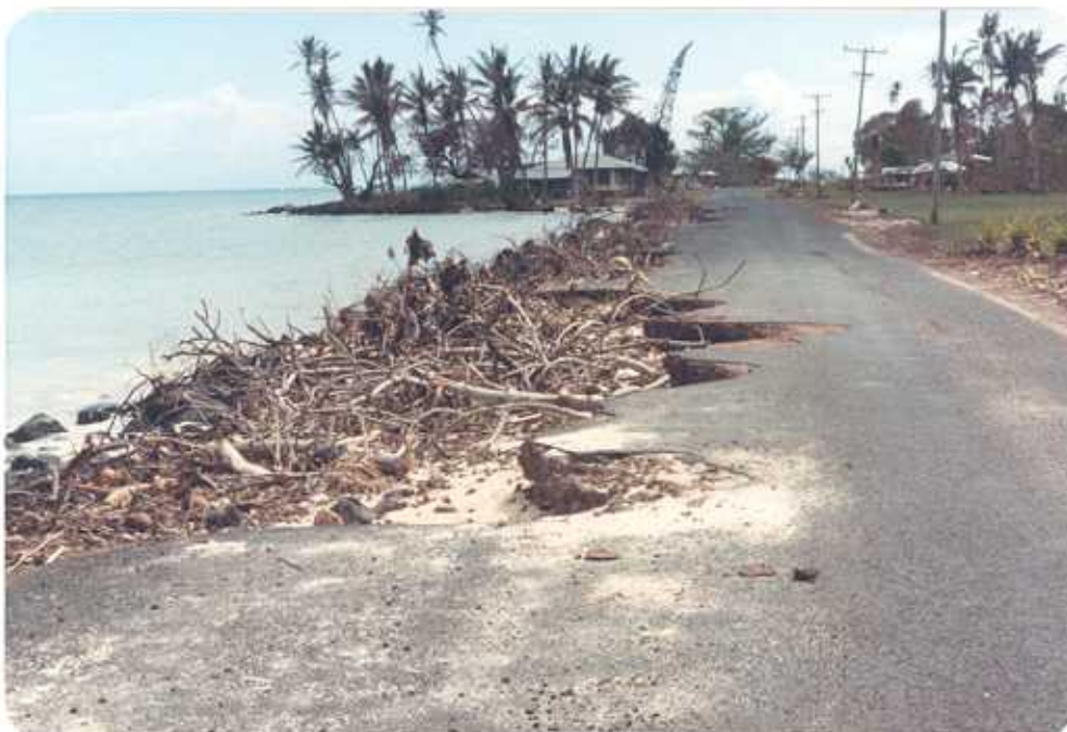
Figure 23. Roads to the west of Apia also suffered considerable damage.
