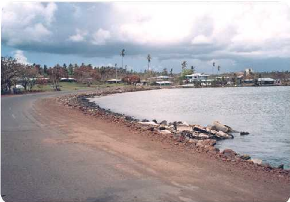
Figure 26. The road at Salcimoa Village lies at the high tide level and even during normal seasonal storms may be awash. Any future increase in sea level will put this area of the coast at high risk from flooding by average tidal fluctuations.
