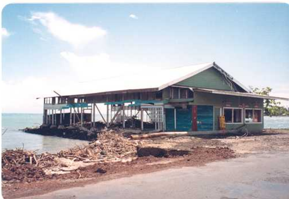
Figure 25. Although roadways suffered damage, some coastal homes on reclaimed land to the west of Apia survived the storm, however the damage sustained was severe in many cases.
