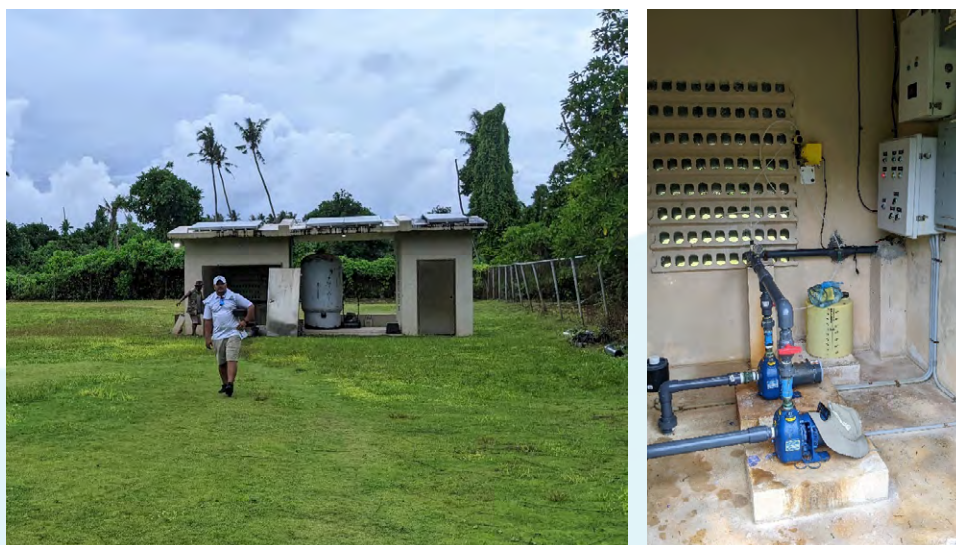
Figure 13. Pumphouse and the two alternating pumps.
