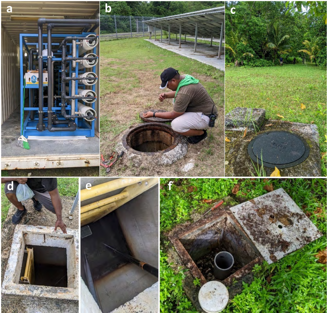
Figure 7. Peleliu pump station and treatment plant: a) reverse osmosis system, b) and c) gallery wells, d) and e) main well, and f) gallery vent.
