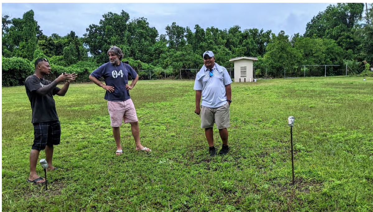
Figure 12. Groundwater catchment area with pumphouse in the background. The two steel poles indicate the edge of the trench that was dug for the two parallel gallery arms to be installed. The trench was then refilled with sands.
