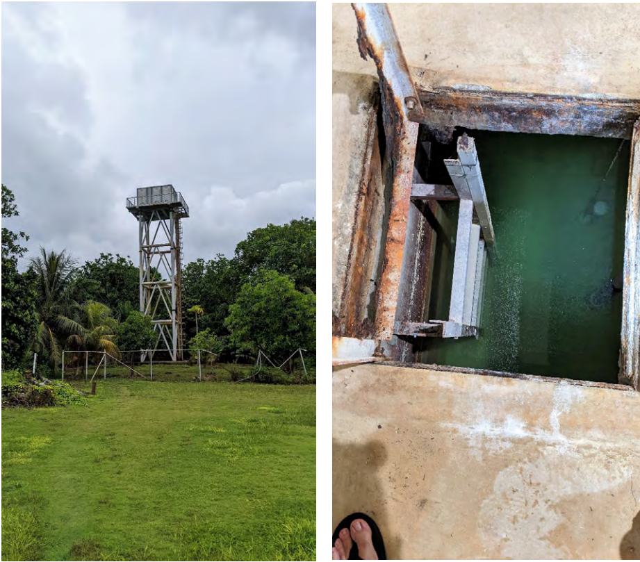
Figure 14. Overhead tank and gallery “well” with damaged lid.
