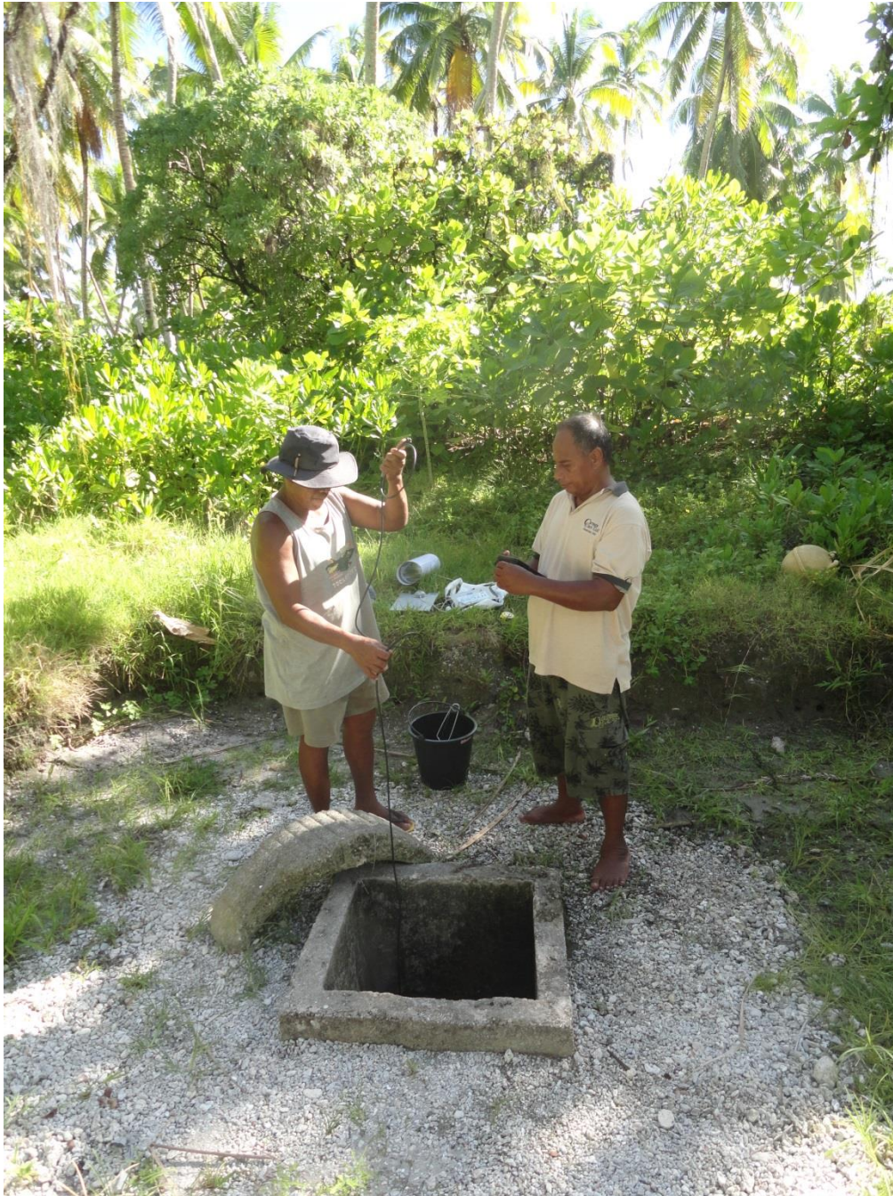
Figure 9. Community well in Kiebu Village assessed by survey team – groundwater from this well is abstracted by bailers (i.e. tins and containers).
