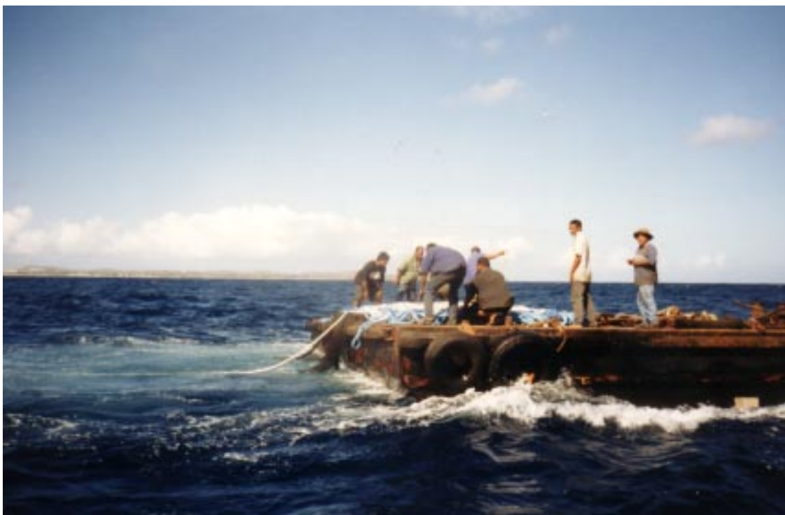
Figure 2: Setting the FAD mooring line at the deployment site
