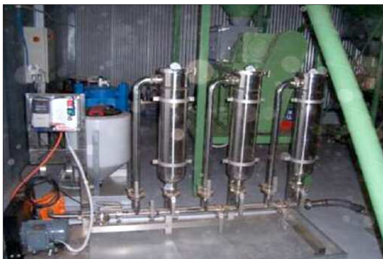
A 5 micron bag filter system
