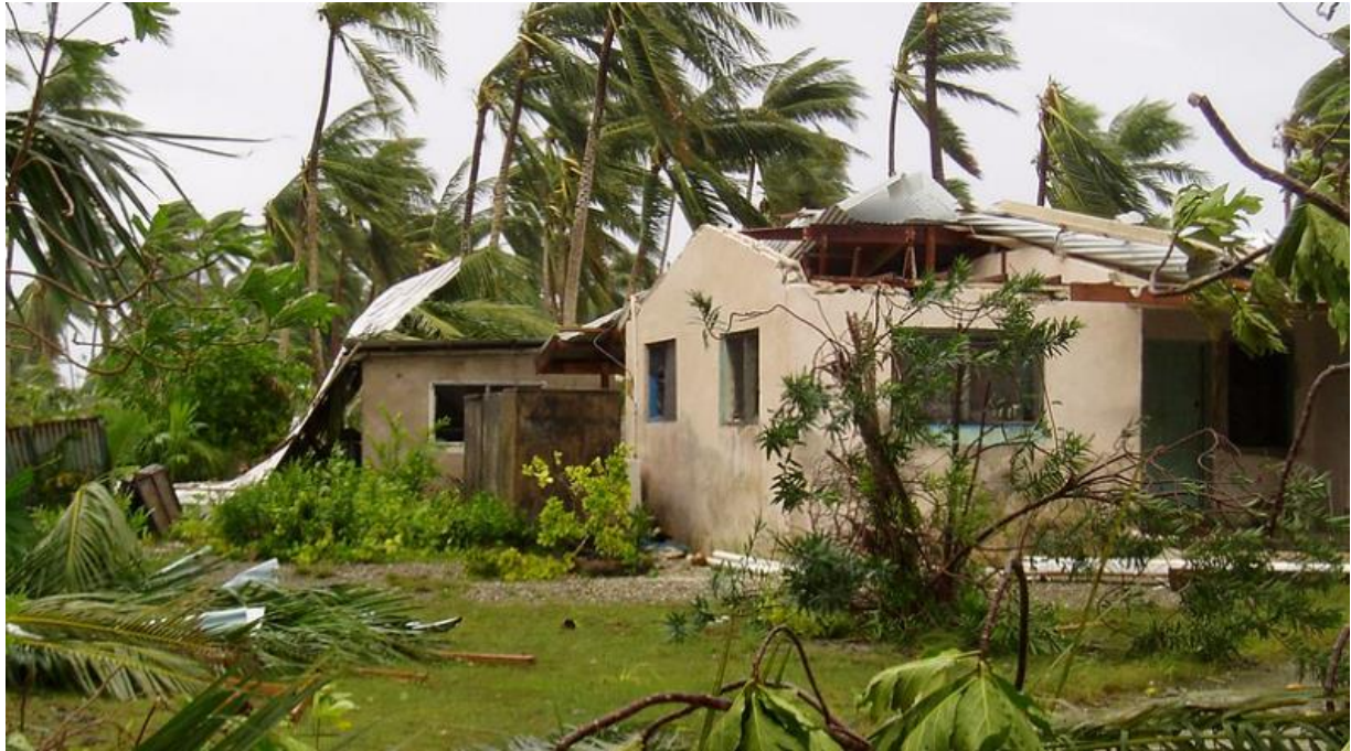
© Damaging winds from Cyclone Percy, Tokelau 2005. Photo: AusAID
