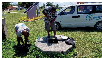
Figure 9. The Jaluit High School well feeds the desalination reverse osmosis unit.
