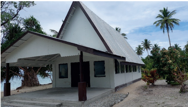
Figure 12. A church on Jaluit islet with new and good roofing, and fascia board, but with no gutters, downpipe or tank.
