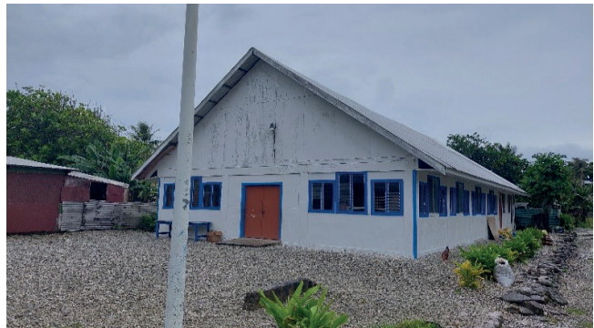
Figure 13. A church on Jabor islet with good roofing and fascia board but with no gutters, downpipe or tanks, which are essential for optimal rainwater harvesting.
