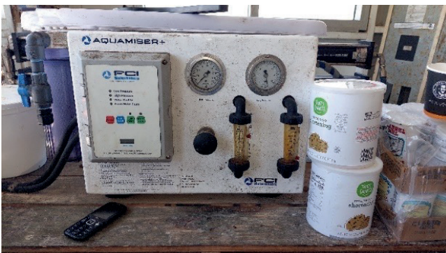
Figure 3. Reverse osmosis desalination unit, Aquamiser+ model, installed at Jaluit High School. It was non-operational during our field mission.
