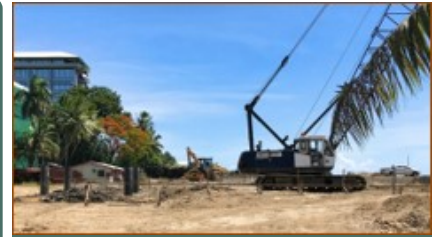
Construction du projet Suva Foreshore, aux Fidji. Image © Pacific Building Solutions
