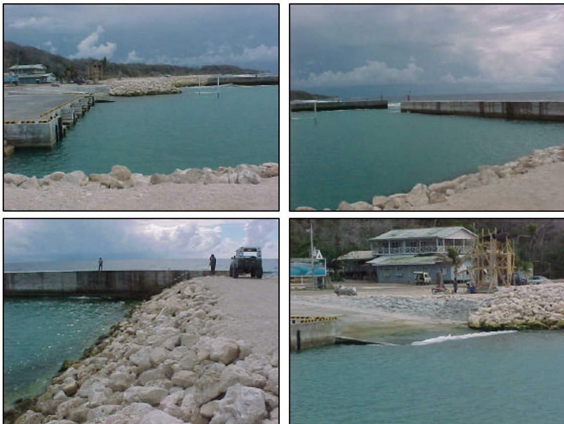
Figure 20. Characteristics of the new harbour facility. Top left – mooring basin/wharf, with quay wall and apron on left of the photo; top right –sub-breakwater and main concrete breakwaters (left and right respectively); lower left – rubble groin, with rip-rap and main concrete breakwater; and lower right – concrete boat ramp, with rip-rap pitched spending slope on the rear right.
