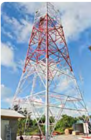
The Betio tower – almost half built
