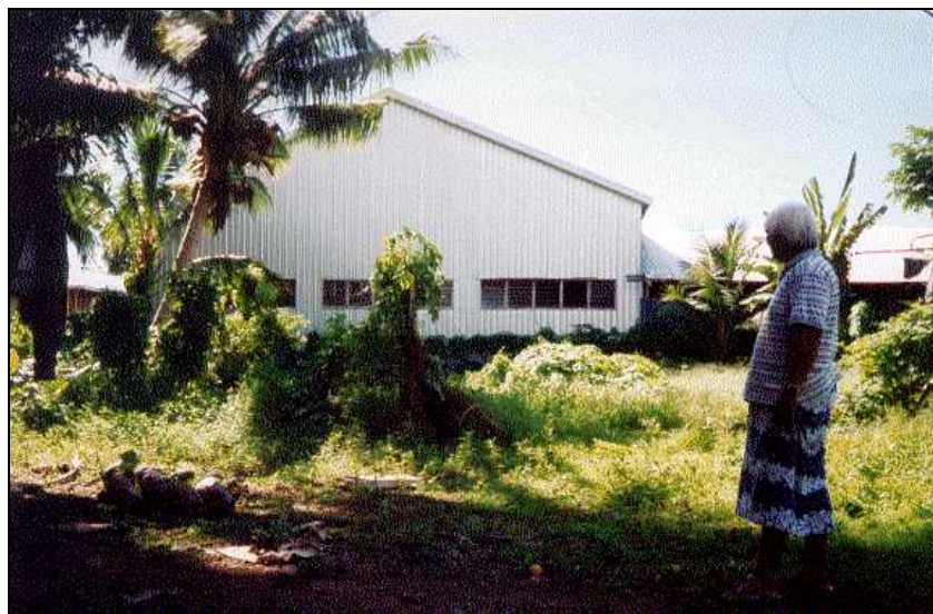
Figure 4.2: Factory situated on reclaimed land, blocking flood channel, Fa'atoia
