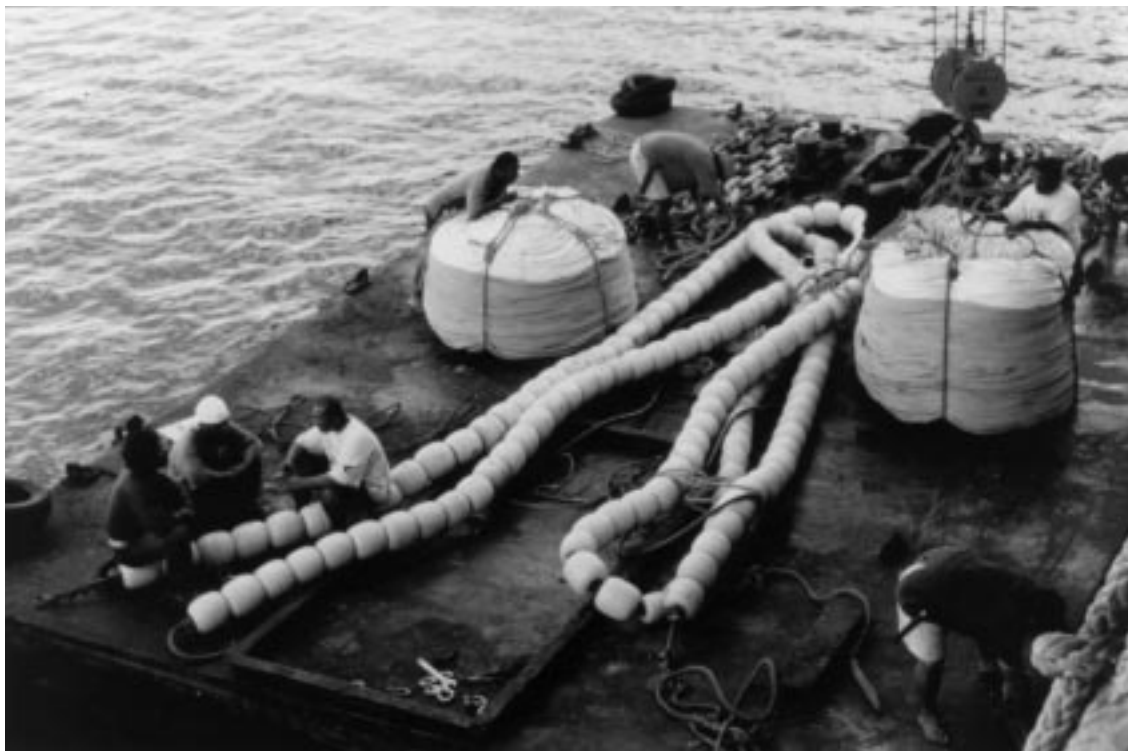
Figure 2: Loading the barge with materials for the two Indian Ocean style FADs
