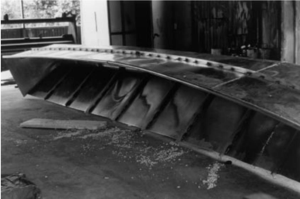
Figure 6: Construction of a hull for a 9.0 m alia catamaran
