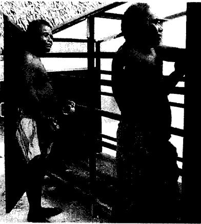
Tarawa, Kiribati: Building a wooden frame for a solar cabinet.
