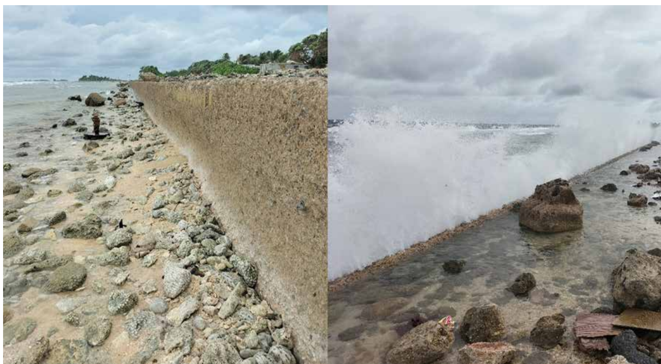
Figure 42: ~80-year-old seawall on Gugeegue islet constructed with local aggregates.
