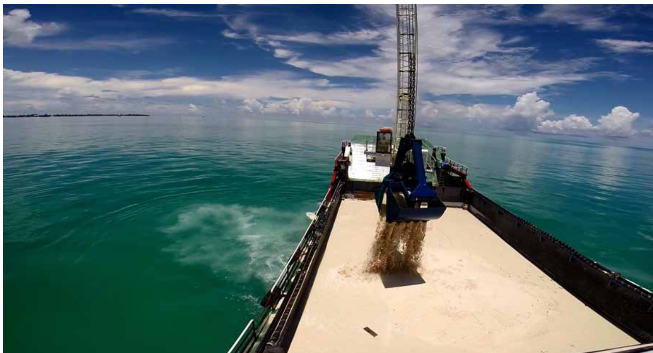
Figure 40: Te Atinimarawa clamshell dredging operation in Tarawa.
