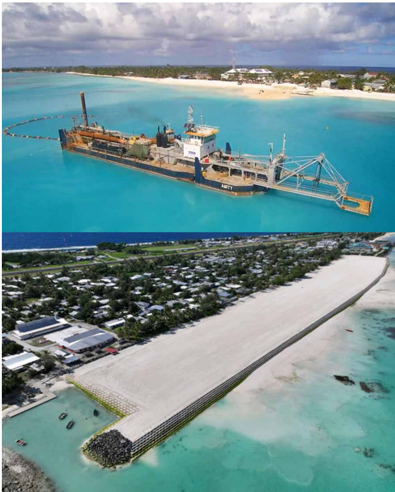
Figure 47: Cutter suction dredge (top) used to complete 6.1 Ha of land reclamation in Funafuti atoll (bottom).
