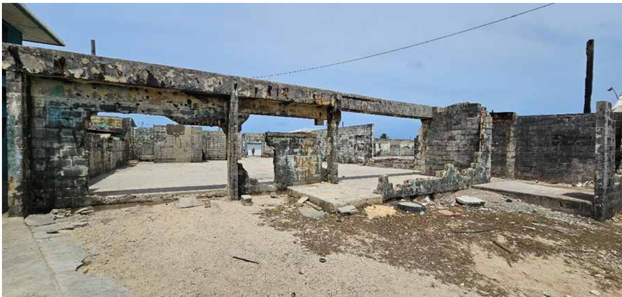
Figure 49: Example of derelict concrete structure on Ebeye, highlighting the potential to recycle concrete.
