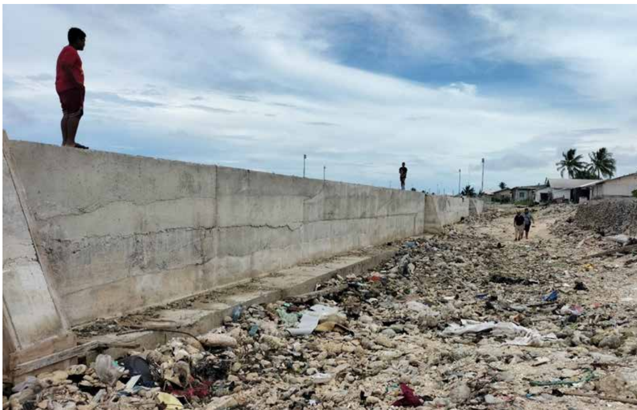
Figure 46: example of a concrete seawall constructed from local sand and gravel resources.
