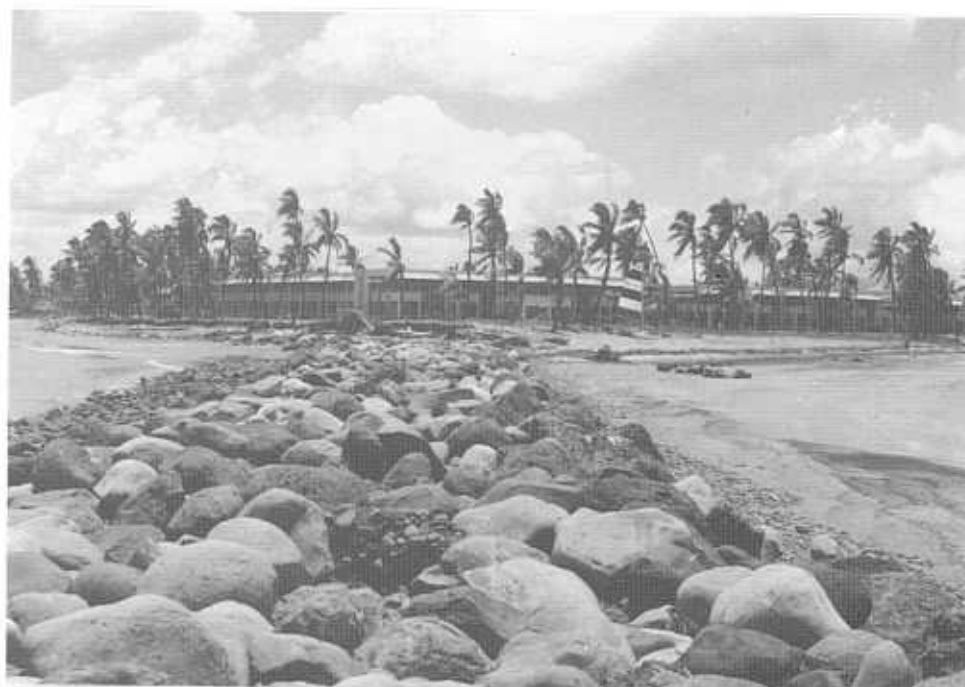
December 1990: Sheraton groyne - after Sina. Note: sand and gravel path is gone.
