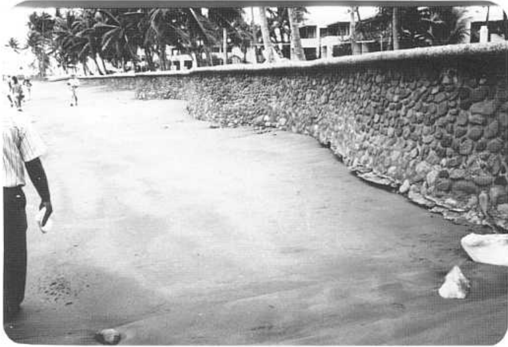
September 1990: Sheraton seawall - before Sina. Note under cutting of wall in foreground.
