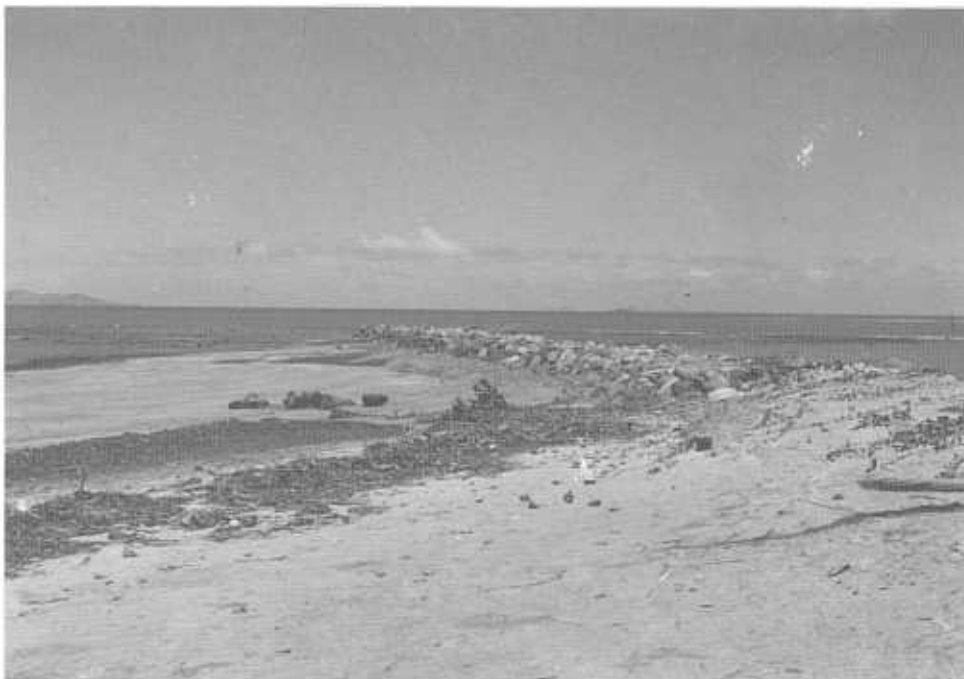
December 1990: Sheraton groyne - after Sina. Note: sand and vegetation scoured.
