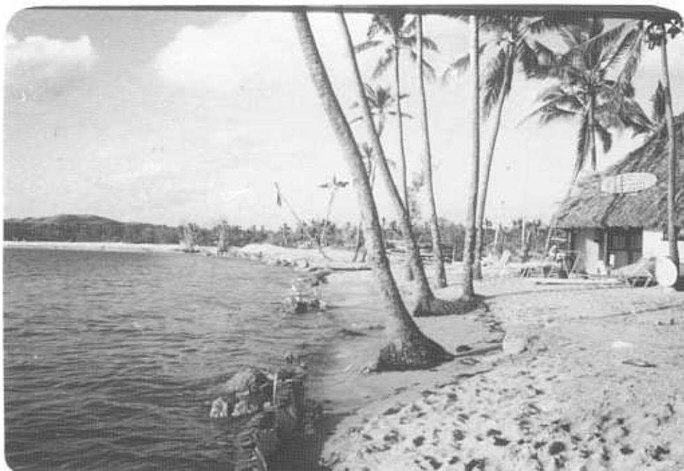
December 1990: Fijian Hotel - after Sina. Note: scouring behind seawall.
