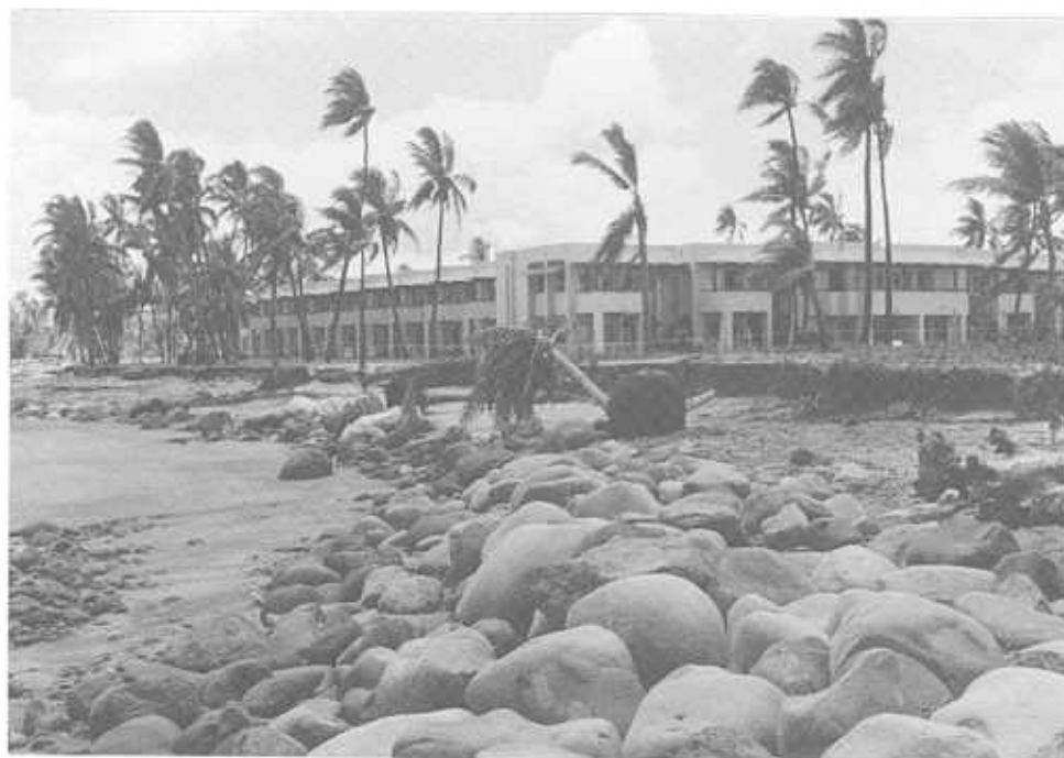
December 1990: Sheraton west side - after Sina. Note: about 10 m of erosion.
