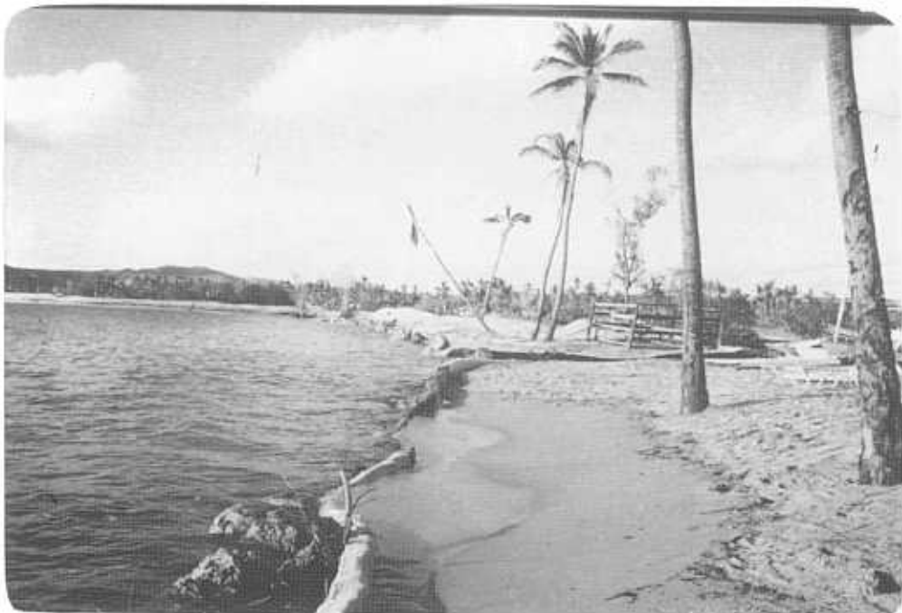
December 1990: Fijian Hotel - after Sina. Note: more scouring behind log seawall.
