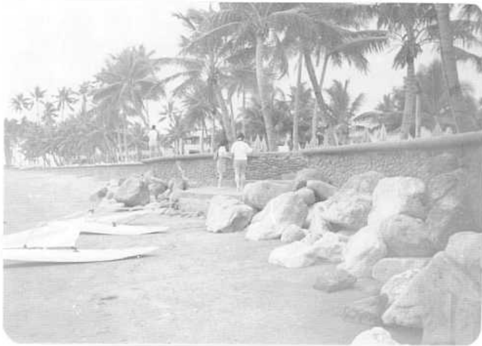
September 1990: Sheraton seawall - before Sina.
