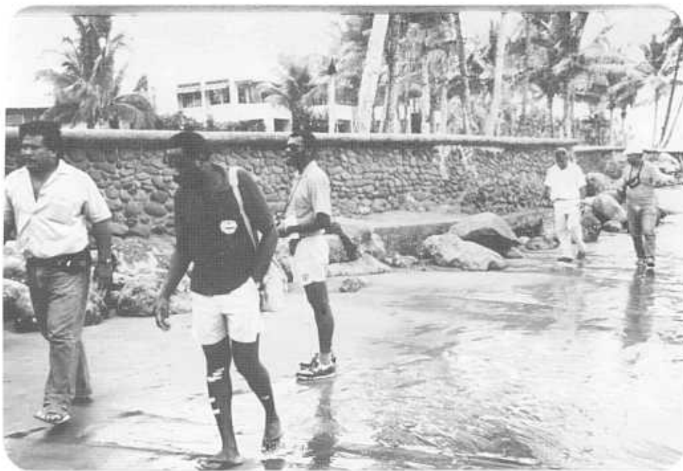
September 1990: Sheraton seawall - before Sina. Note: concrete slab toe protection in front of wall.
