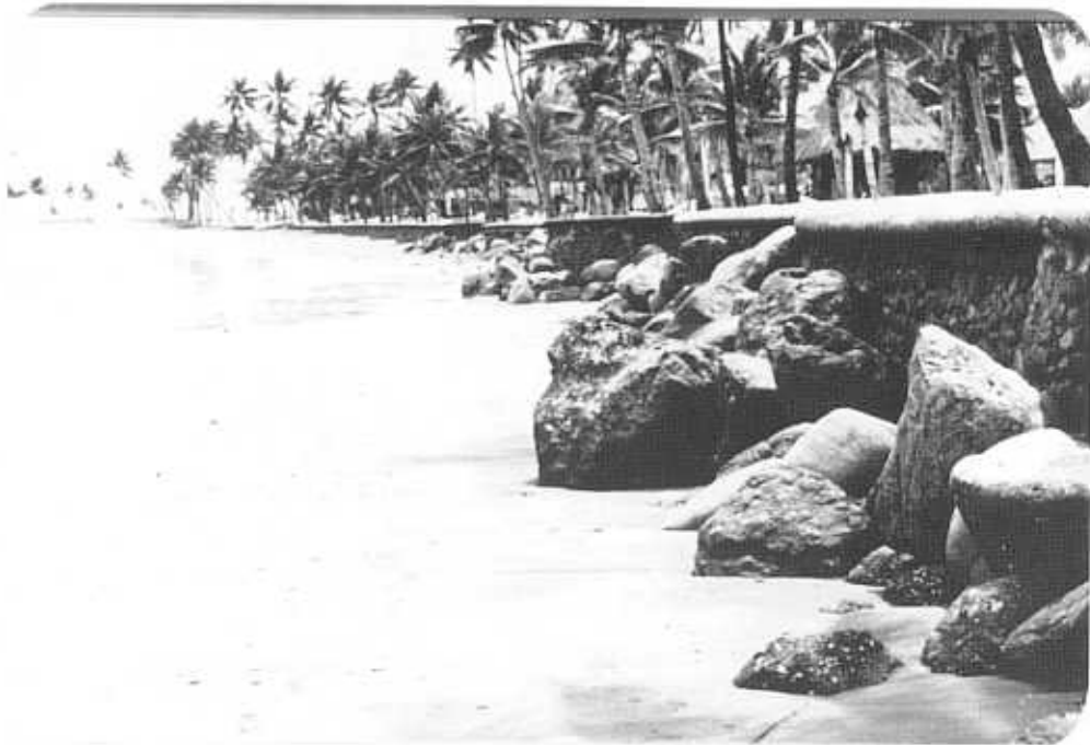
September 1990: Sheraton seawall before Sina.
