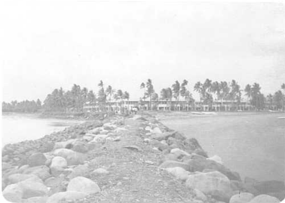
September 1990: Sheraton groyne - before Sina. Note: sand and gravel path on top of groyne.
