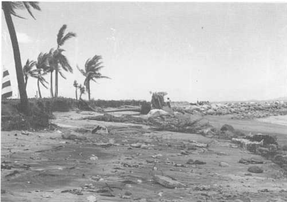
December 1990: Sheraton west side - after Sina. Note: rubble mound protection is gone.
