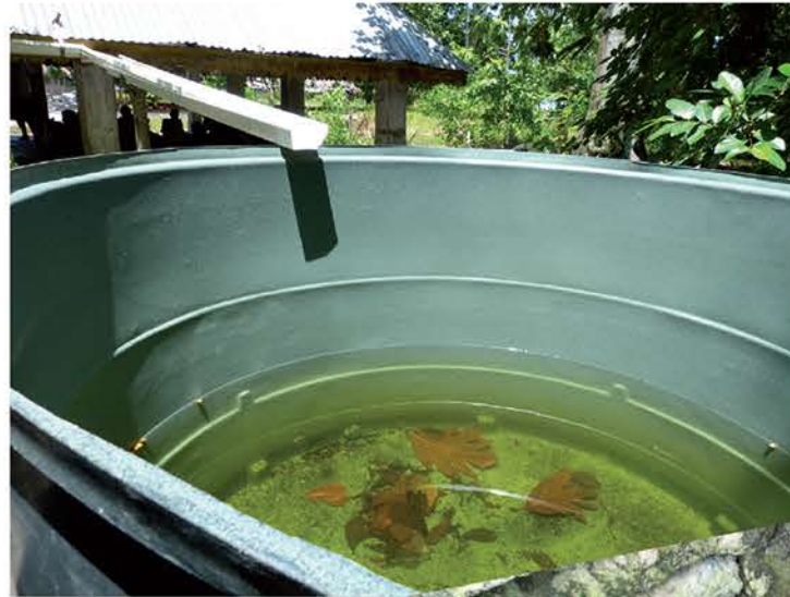
Unprotected rainwater tank, Carlo Iacovino, SPREP 2013
