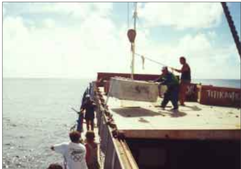
Figure 5: Deploying the FAD anchor block in Rarotonga from M/V Manu Nui [Photo: Steve Beverly]
