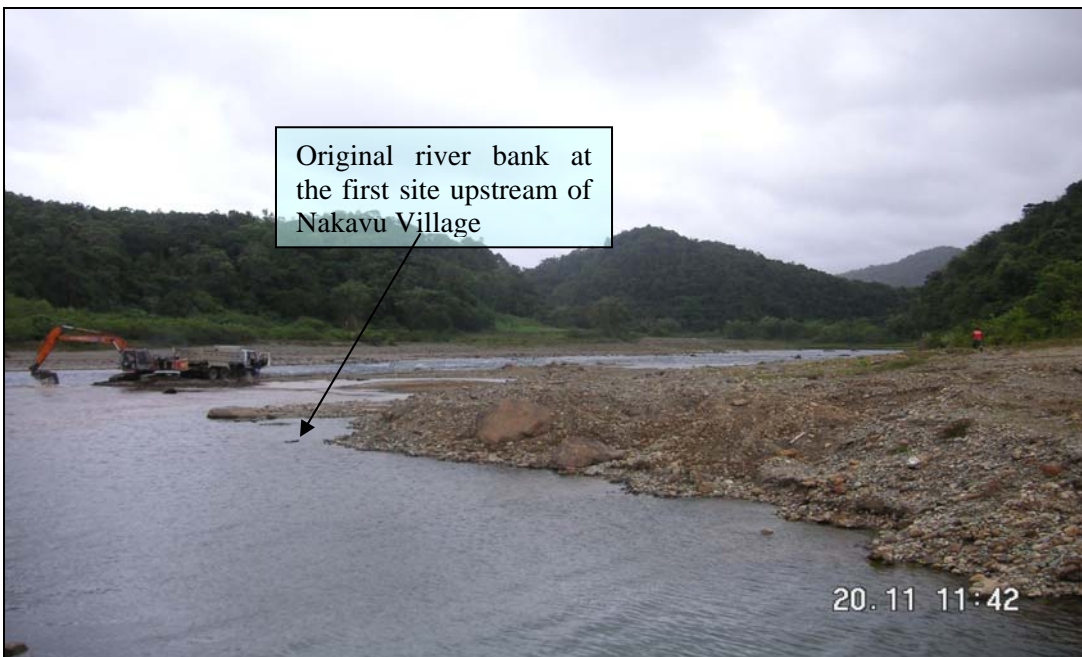
Figure 8. River bank at Nakavu Village begins to erode and widen due to the impact of extraction upstream of the village.
