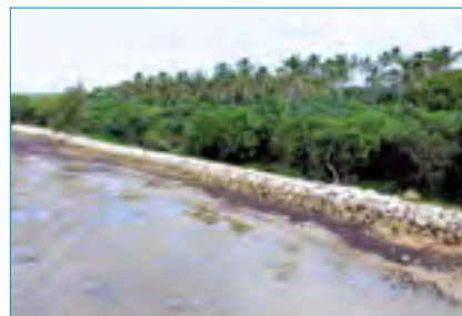
Completed rock revetment at Kanokupolu, Tonga
