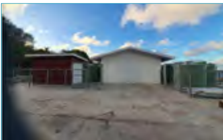
New water facility building, Banaba Island, Kiribati
