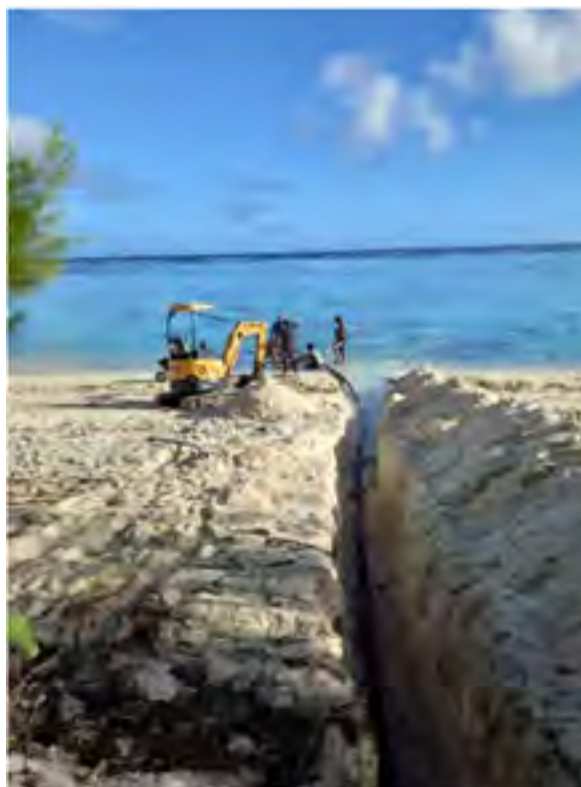
Installing the saltwater intake
