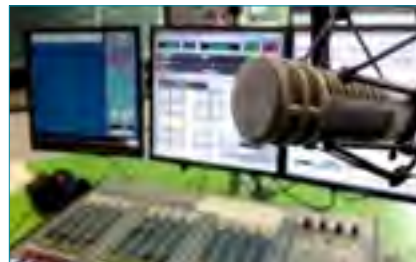
Newly equipped national radio station with capacity to broadcast Eco-Paradise FM throughout Palau
