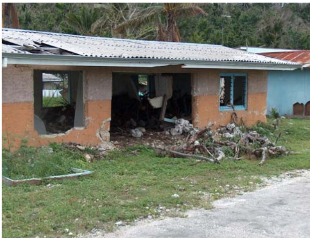
Figure 3: Building in Makefu smashed by coral rubble and tree debris.
