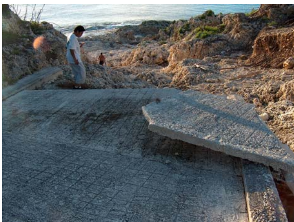
Figure 8: After the sealing was removed, waves dug huge holes in the weakly cemented fill: Uluvehi (above) and Namakulu (below) sea track.
