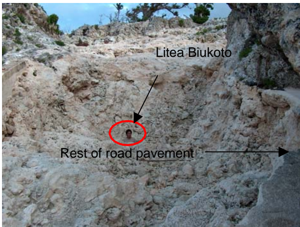
Figure 8: After the sealing was removed, waves dug huge holes in the weakly cemented fill: Uluvehi (above) and Namakulu (below) sea track.
