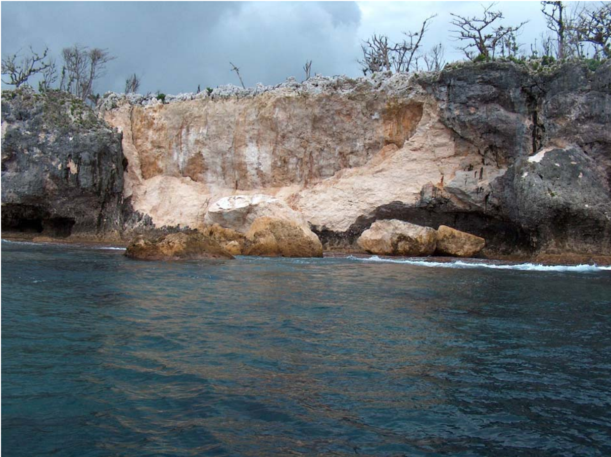
Figure 1: Cliff failure at Makefu South – one of the biggest failures that occurred during TC Heta.
