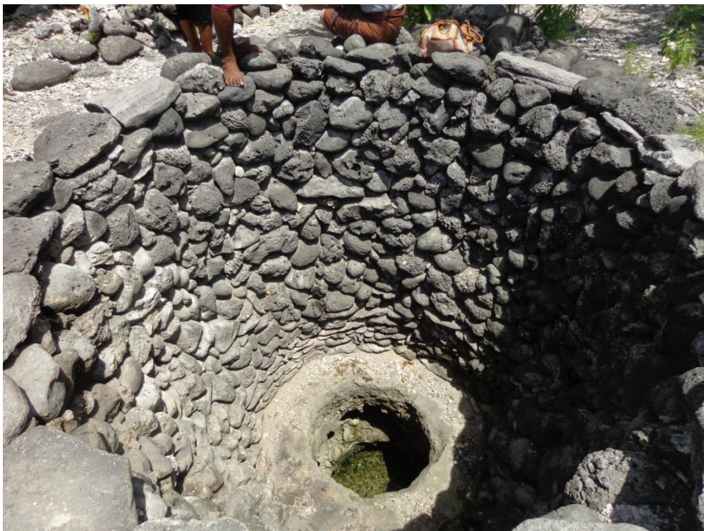
Figure 9. Typical household well excavated down to bedrock and using coral rock as casing materials, without parapet and fence.
