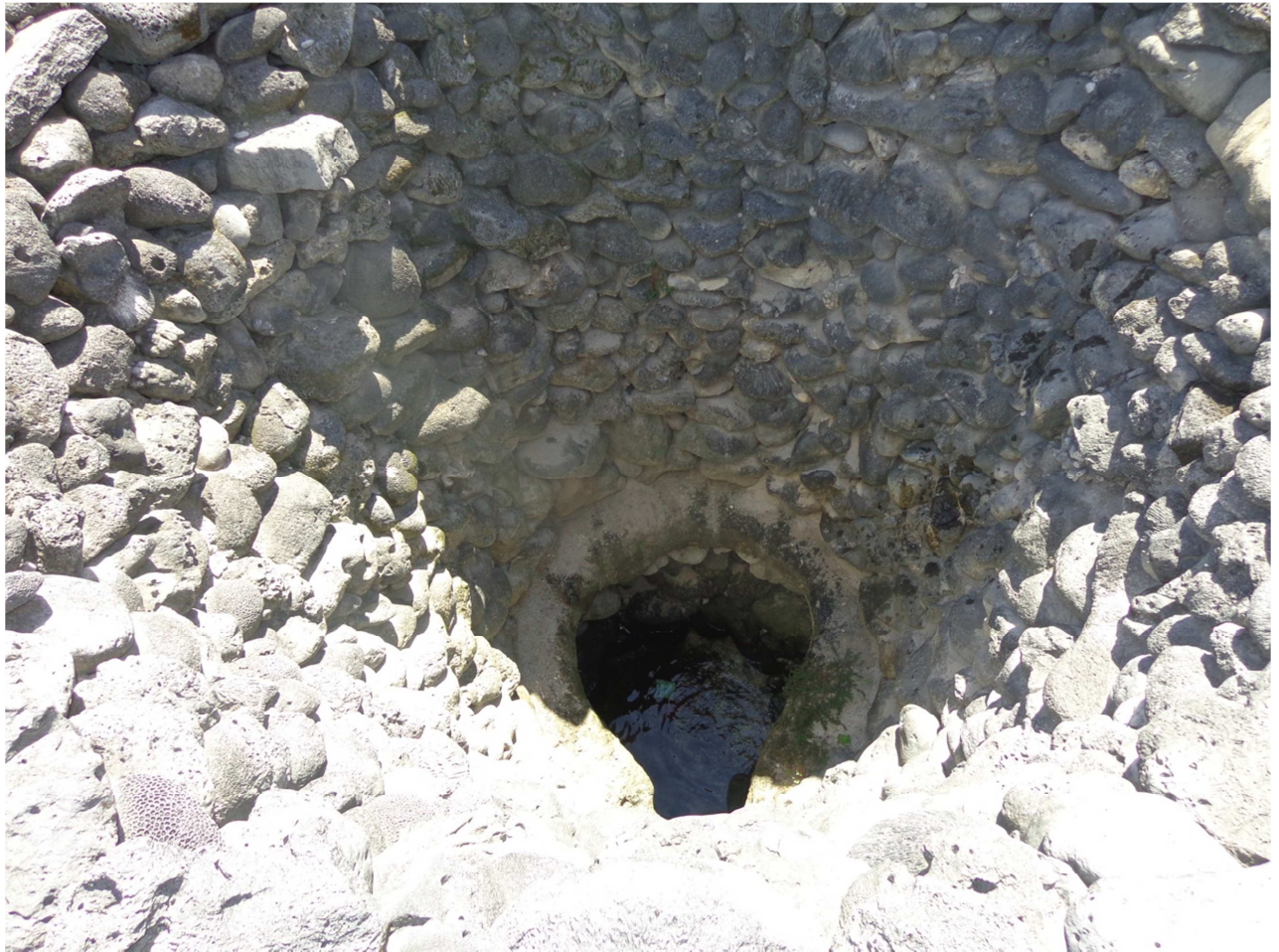
Figure A11-1. A household well using coral rock as casing material right down to bedrock.
