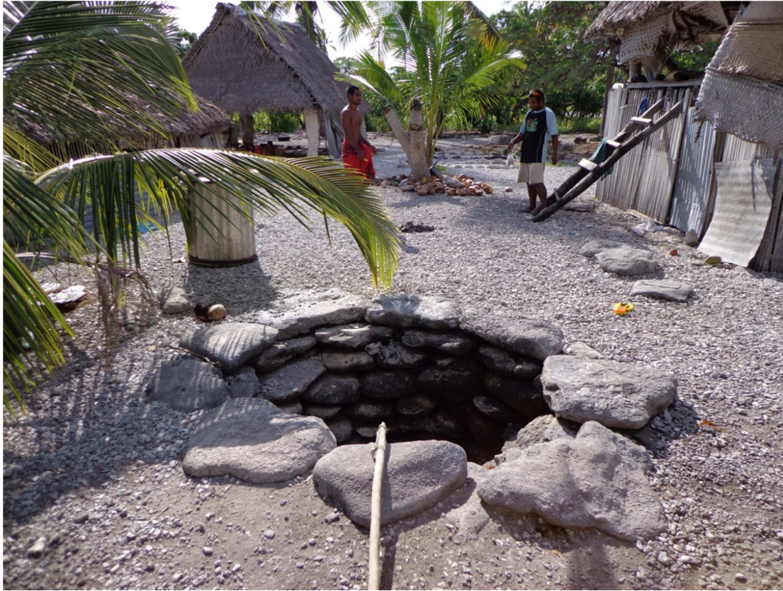
Figure A11-6. Tamana distribution line from a poorly protected household well.
