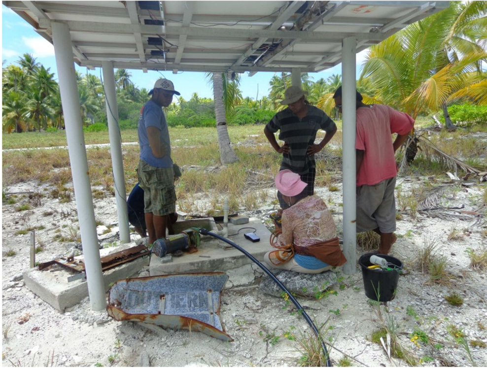
Figure A11-4. Survey team assessing the Muribenua Village well; water is abstracted by solar pump.
