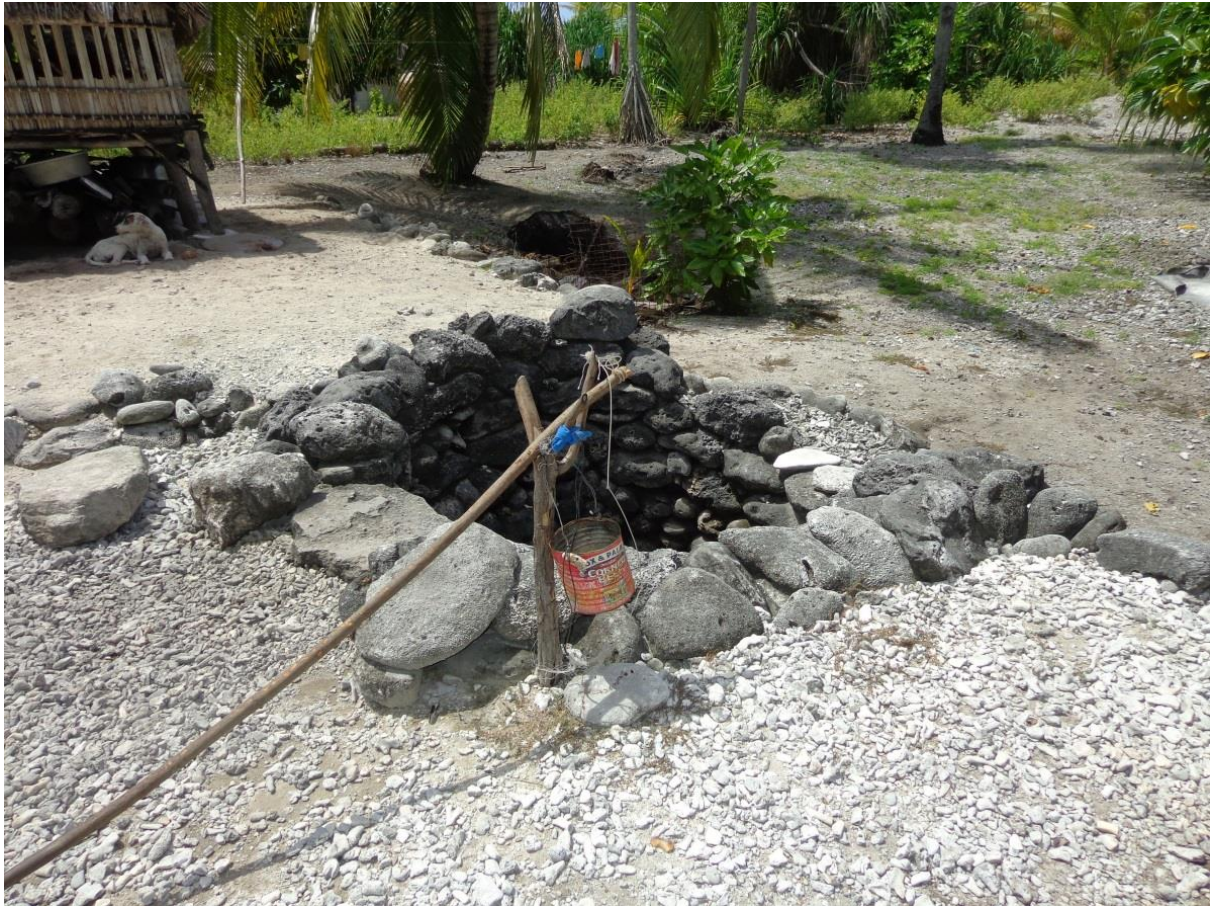
Figure 10. Typical bailer used for abstraction of groundwater from a local well, Nikumanu, Nikunau.
