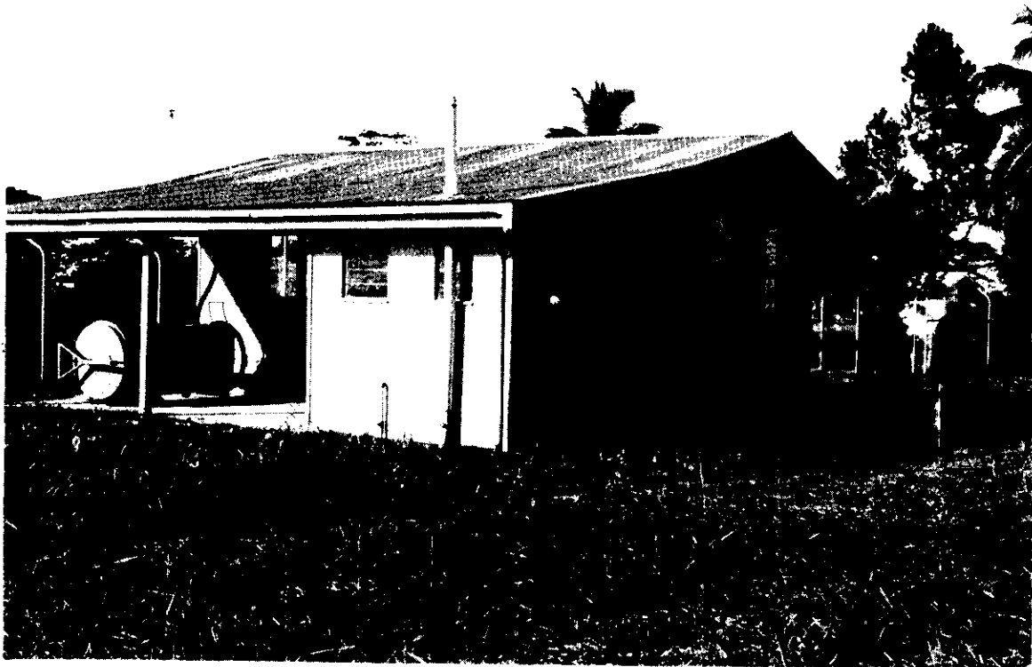
Laboratory building within the Koronivia Post-Entry Quarantine Station showing location of fumigation chamber.
