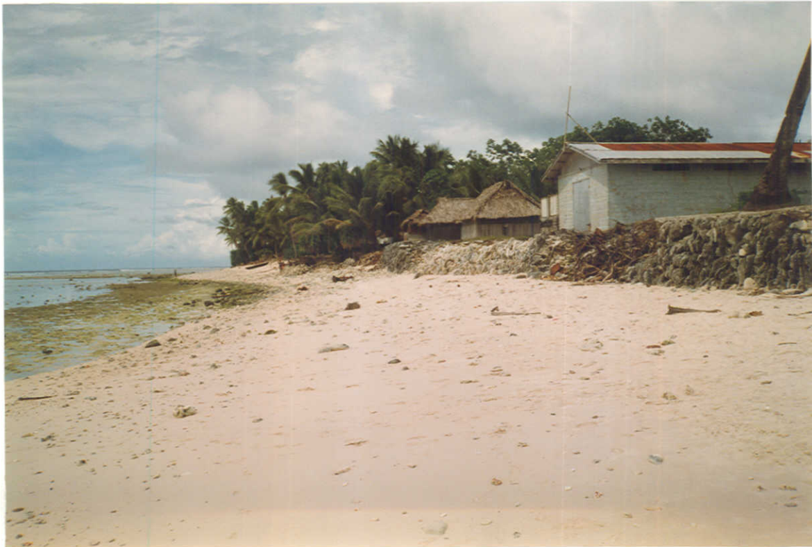
Figure 11. Rawannawi, Marakei. View north (at location of reef passage) along shoreline showing protection response with locally constructed, near vertical seawalls.
