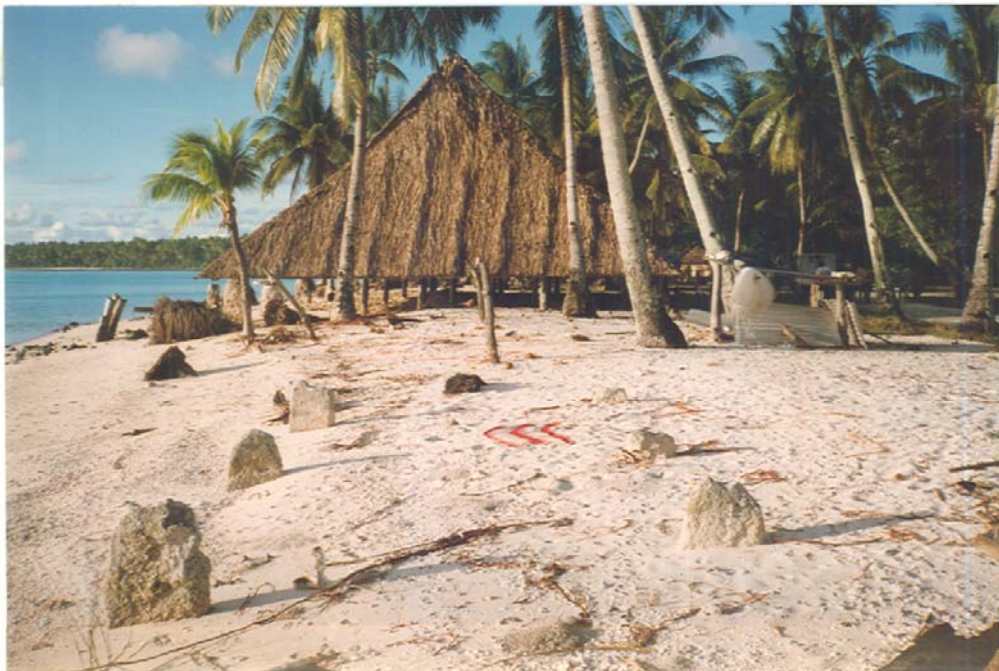
Figure 9. Tebunginako, Abaiang. View northwest showing erosion extending beneath maneaba. The maneaba is no longer used because the floor is flooded during westerly seas and high tides. The remaining foundation blocks of an abandoned building are visible in the foreground at the level of normal high water.
