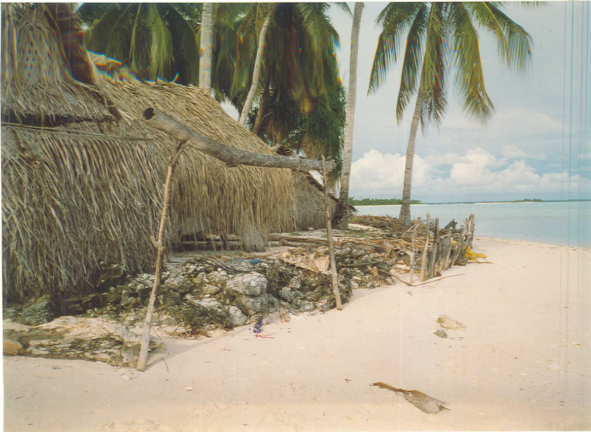
Figure 45. Takaeang, Aranuka. View of remaining gabion basket seawall in front of teacher's quarters near school.
