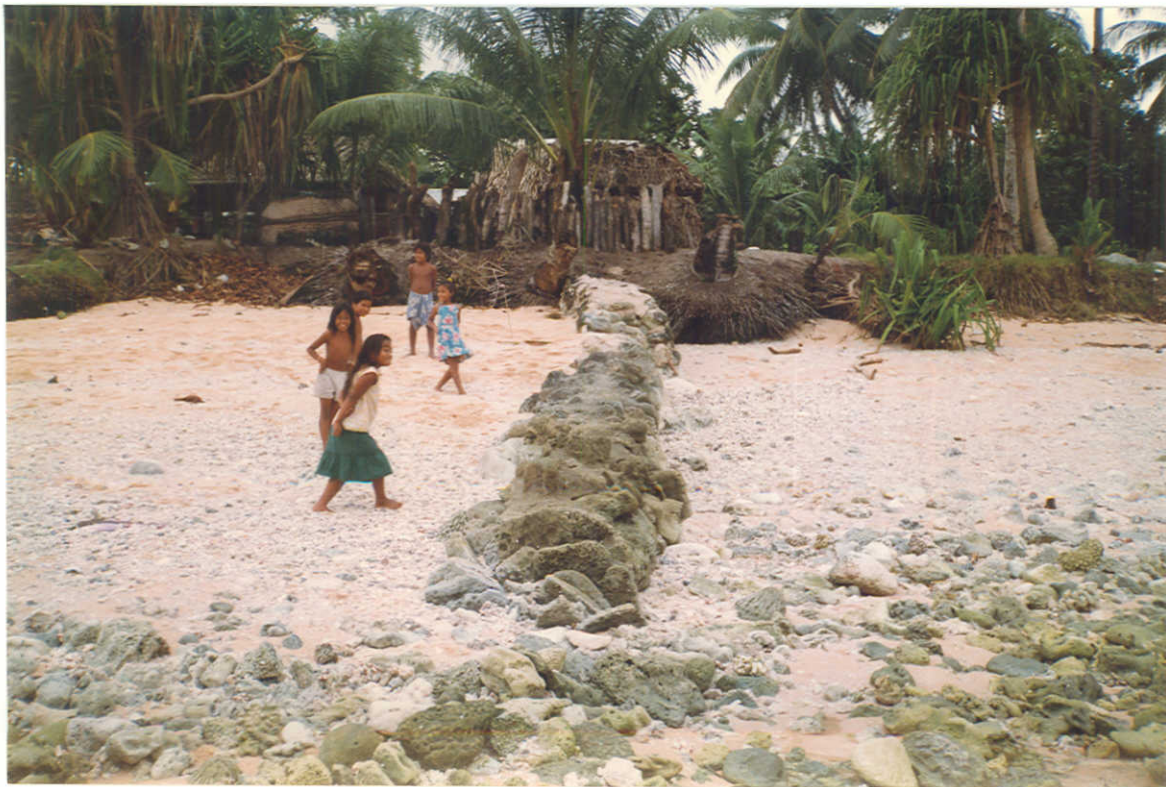
Figure 18. Naka Primary School, Makin. View of locally constructed small groyne located approximately 200 m south of school site. The greater volume of sand on the left (north side) of the groyne indicates that the most recent predominant direction of longshore transport has been from the left (north).
