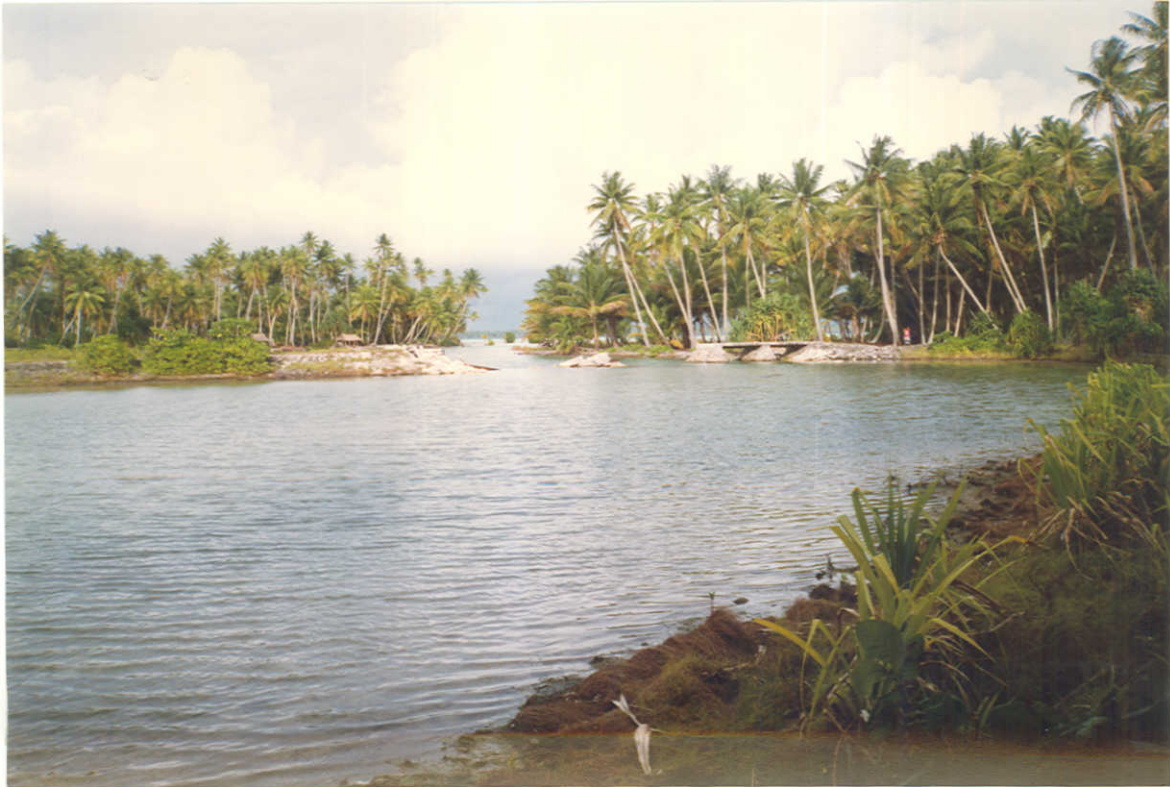
Figure 14. Baretoa Passage, Marakei. View east through passage past abandoned causeway and towards lagoon. Since closure of the passage the causeway has been partially removed in an attempt to restore the natural flow and re-open the passage.
