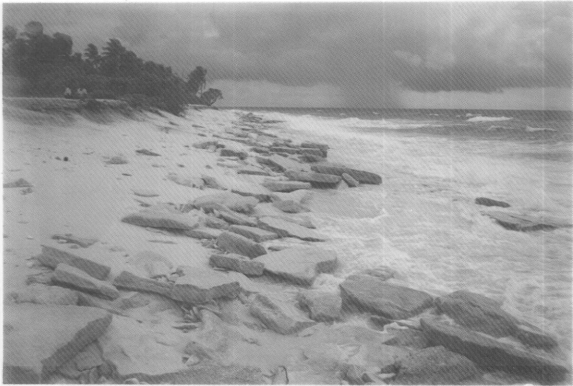
Figure 29. West end of airfield runway, north of Barebuke, Tamana. View south showing erosion scarp at left and scattered slabs of broken beachrock.
