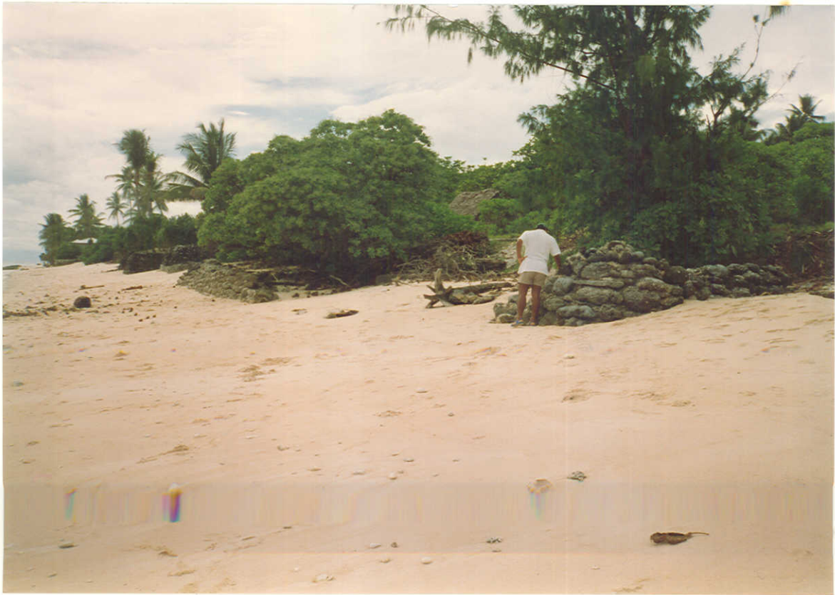
Figure 42. Tabomatang, Nikunau. View northwest at location of beach profile site showing remains of seawall on upper foreshore.
