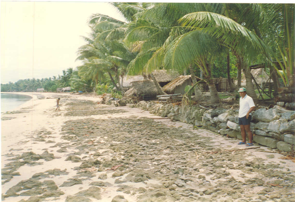
Figure 48. Buariki South, Aranuka. View north at beach profile site showing exposed beachrock in front of seawall constructed of beachrock slabs quarried from the lower foreshore. Note absence of any beach sediment on upper foreshore.
