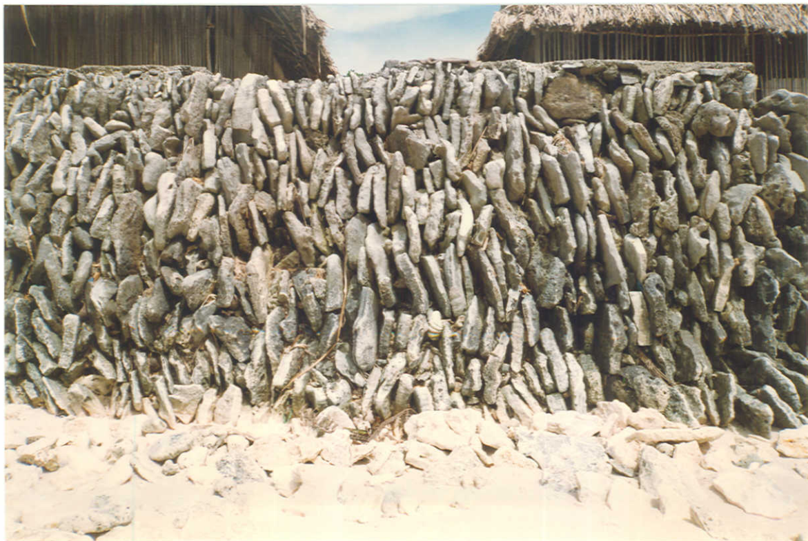
Figure 12. Rawannawi, Marakei. View of near vertical seawall constructed of tabular coral and beachrock slabs. The wall is over two metres high.
