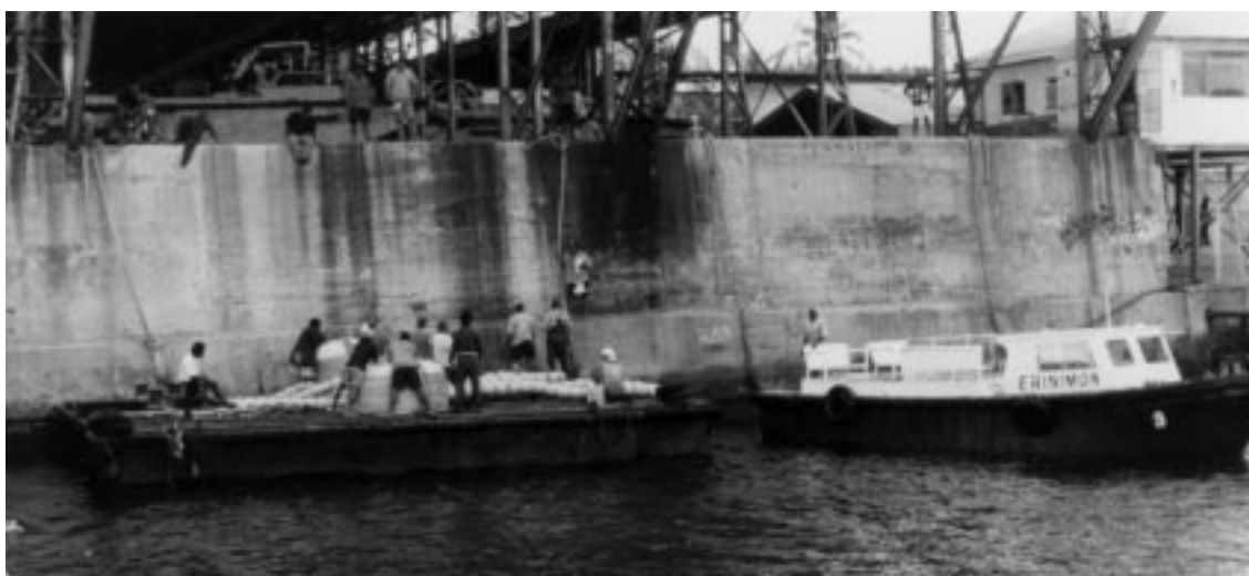
Figure 3: M/V Erinimon ready to tow the barge to the deployment sites
