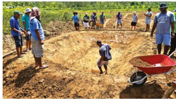
Putting the finishing touches to our hand-dug, household-scale fish pond by planting grasses on the dykes.
