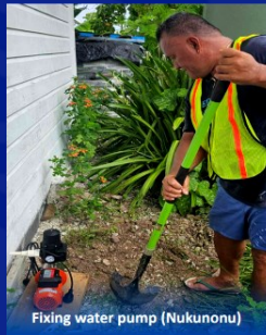
Fixing water pump (Nukunonu)
