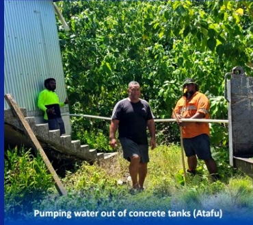
Pumping water out of concrete tanks (Atafu)
