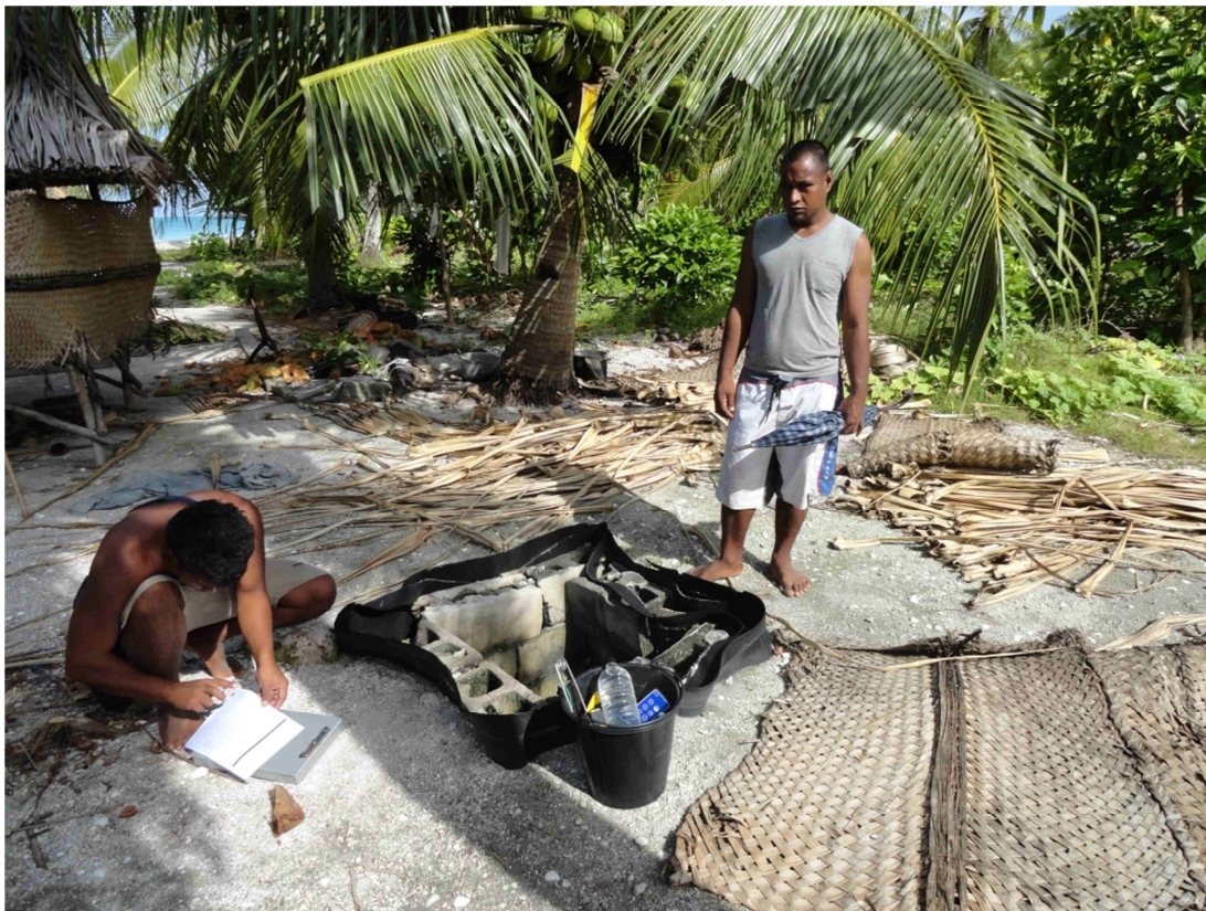
Figure A12-8. Household well using concrete blocks as casing material, with no apron.
