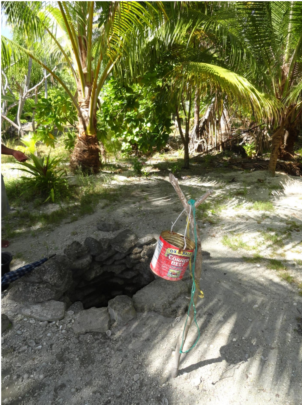
Figure 9. Typical bailer used for abstraction of groundwater from a local well, Aonobuaka, Abaiang.
