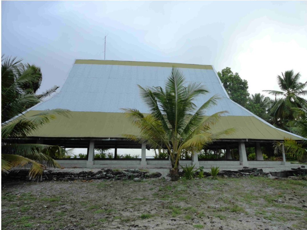
Figure A12-13. A maneaba at St Joseph College – representing a potential RWH centre.
