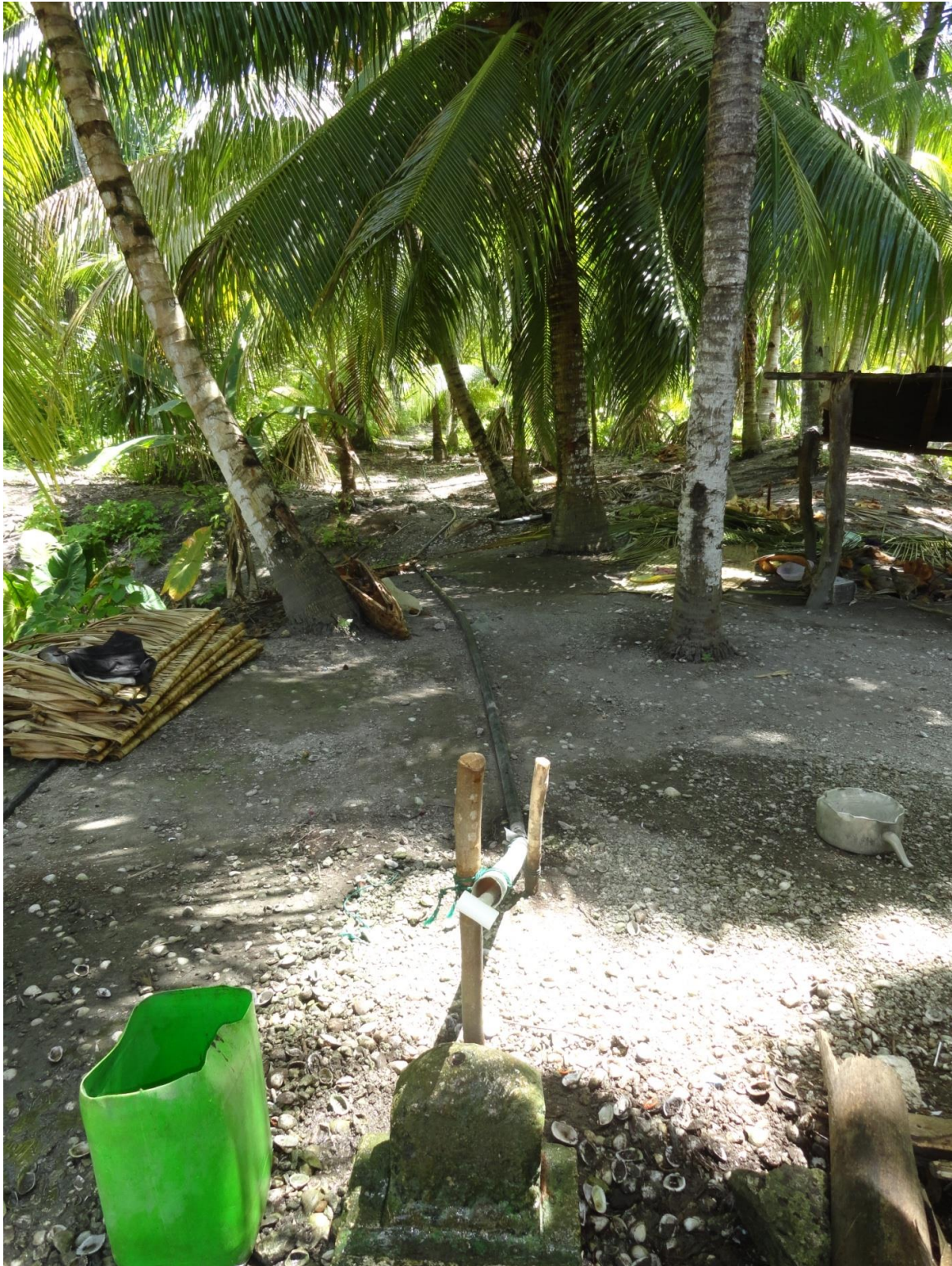
Figure 10. Kiribati hand pump used for abstraction of groundwater from a distant local well, Ewena, Abaiang.
