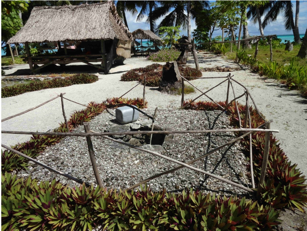
Figure A12-17. Household well in Taniau showing coral rock casing, coral gravel parapet, and the use of the Tamana pump, with the distribution line resting on a plastic container.
