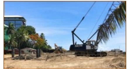
Construction of the Suva Foreshore Project, Fiji. Image © Pacific Building Solutions
