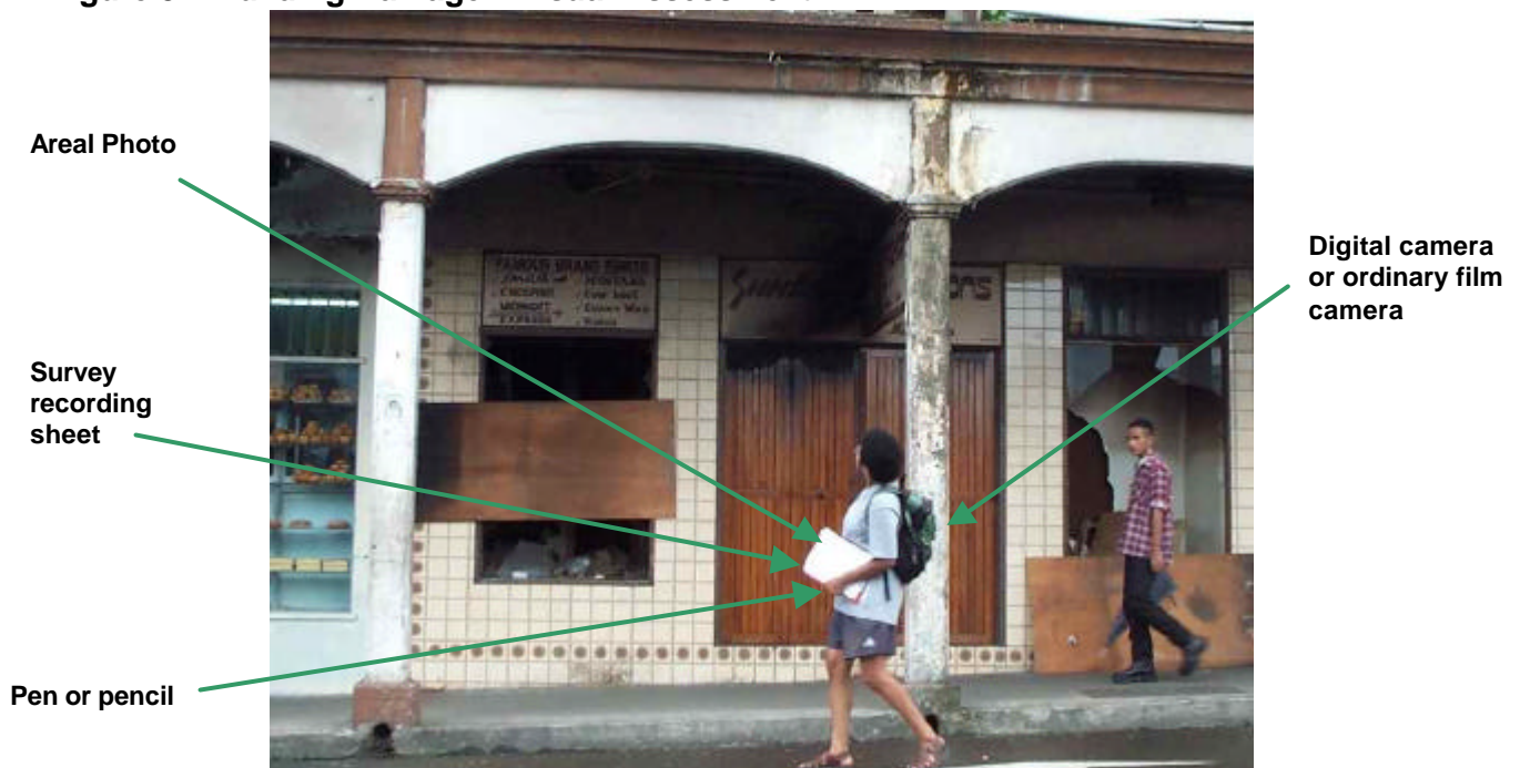
Figure 3. Building Damage – Visual Assessment
