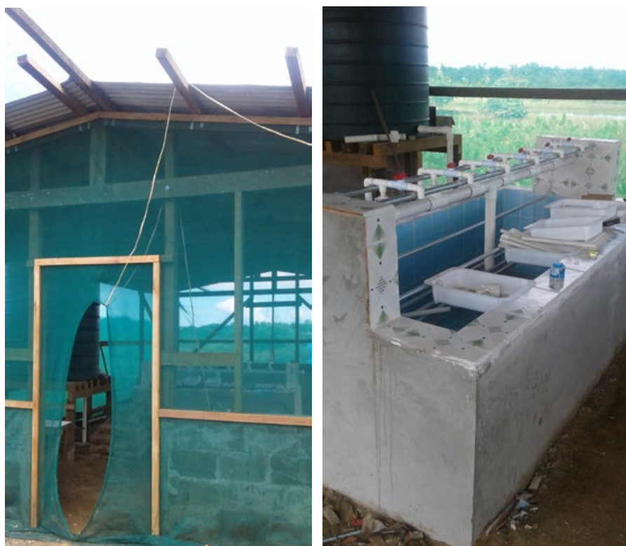
Figure 2. Tilapia hatchery under construction at Katarina's farm.
