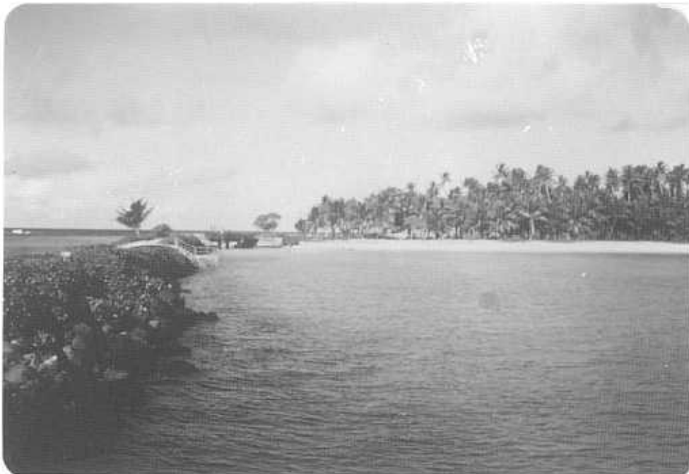
Figure 8. Oinafa Wharf: south side of causeway showing bridge at landward end of causeway.
