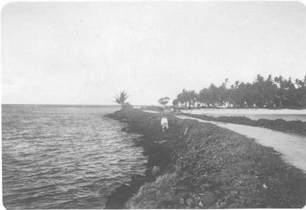
Figure 7. Oinafa Wharf: north side of causeway showing armour stone sizes.
