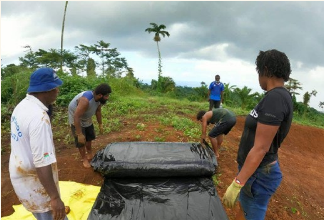
Josephine and colleagues laying the pond liners. © Josephine Rambay
