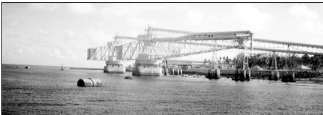
Figure 3: Mooring buoys used for tying up bulk carriers when loading phosphate
