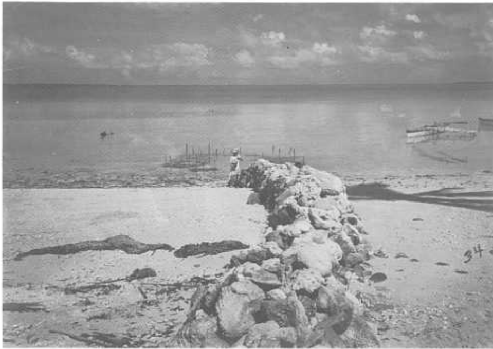
Figure 7. Groyne in front of Tebunginako maneaba, facing west. Note accumulation of material on the left (south) side and depletion of material on the right (north) side.
