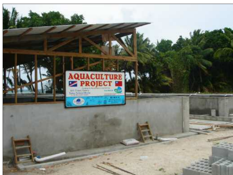
Taiwanese marine fish hatchery under construction
