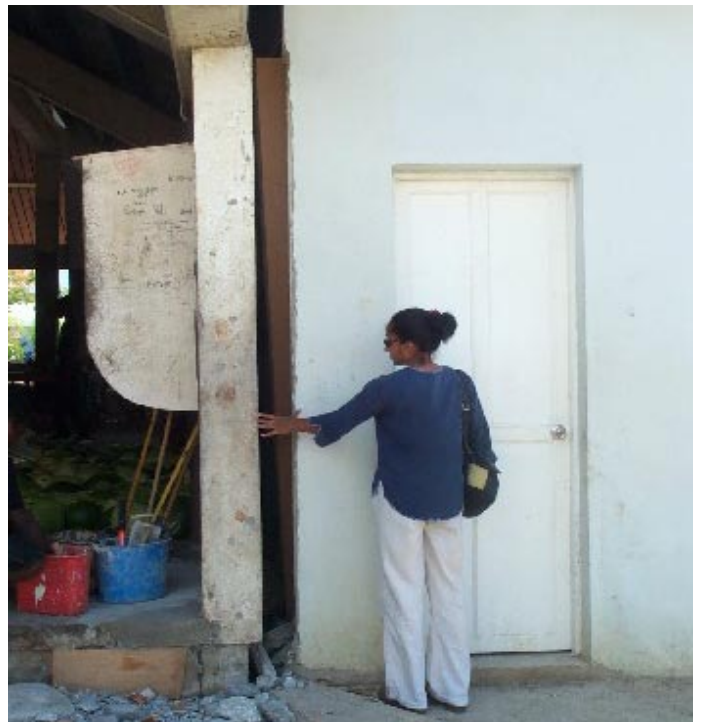
Figure 28: Detached Market toilet block.
