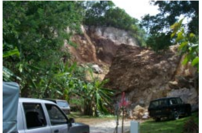
Figure 42: Toppling failure from the cliff face near Pango Resort.
