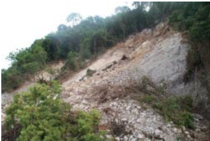
Figure 40: Massive slope failure in tuff above Star Wharf access road.
