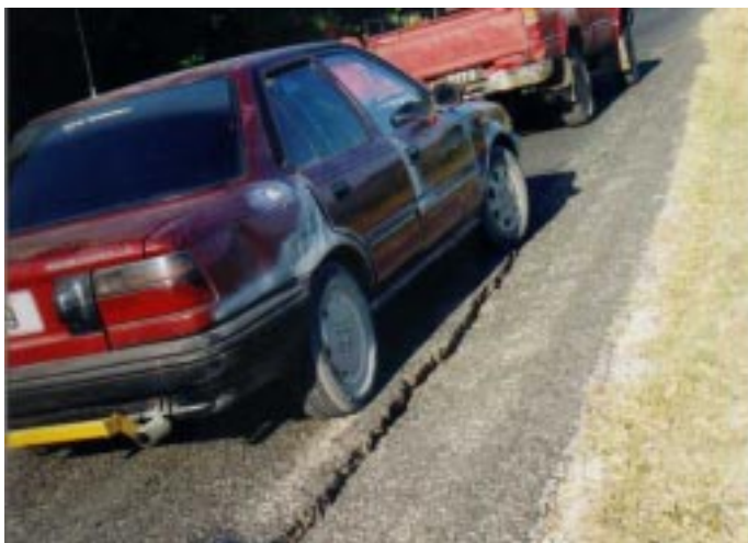
Figure 41: Road embankment collapse, Star Wharf road.
