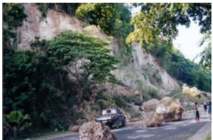
Figure 38: Blockage of Star Wharf access road by landslide.
