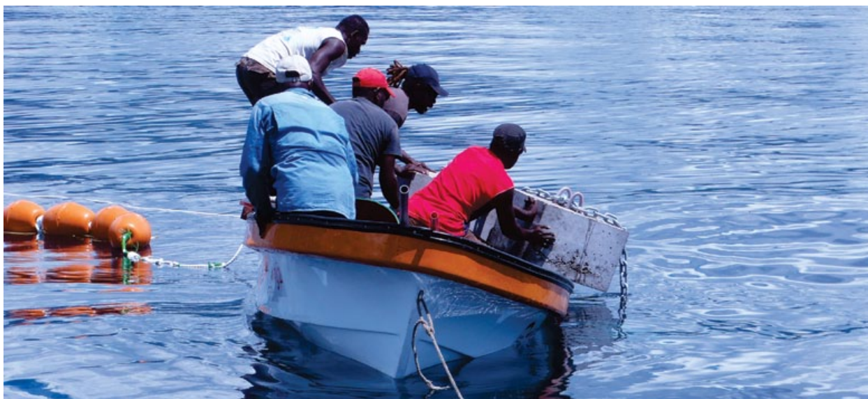
Figure 9. Cement block anchor about to be deployed.
