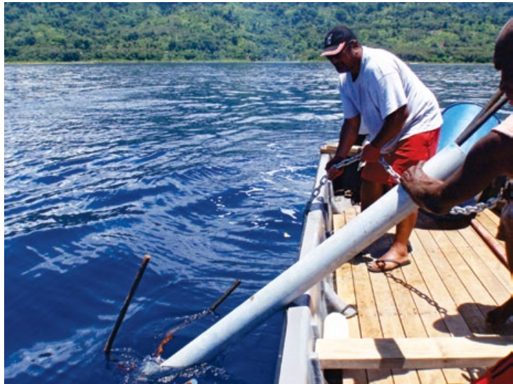
Figure 2. Deploying a nearshore surface FAD from a 23 ft open Yamaha banana boat using a grapnel for anchor.
