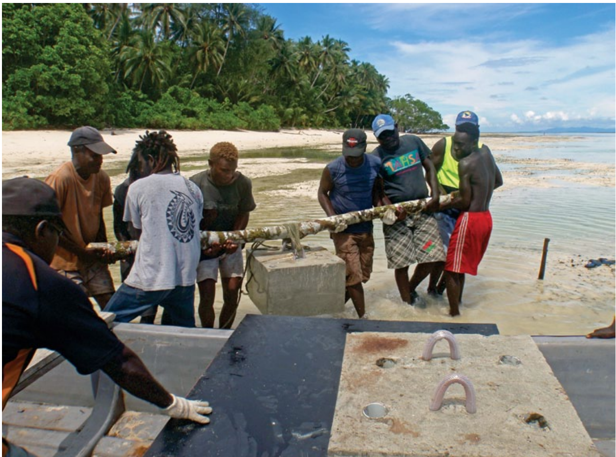
Figure 6. Loading a cement block on to the deployment vessel.
