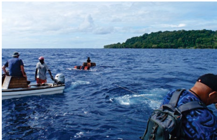
Figure 3. Using two boats to tow a bulk anchor to the deployment site.
